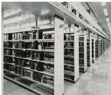
Multi-tier bookstacks and mezzanine cellular decking installed in September, 1964 at University of Victoria, B.C. Mr. Dean W. Halliwell, Chief Librarian. R. W. Siddall Associates, Victoria, B.C., Architect
