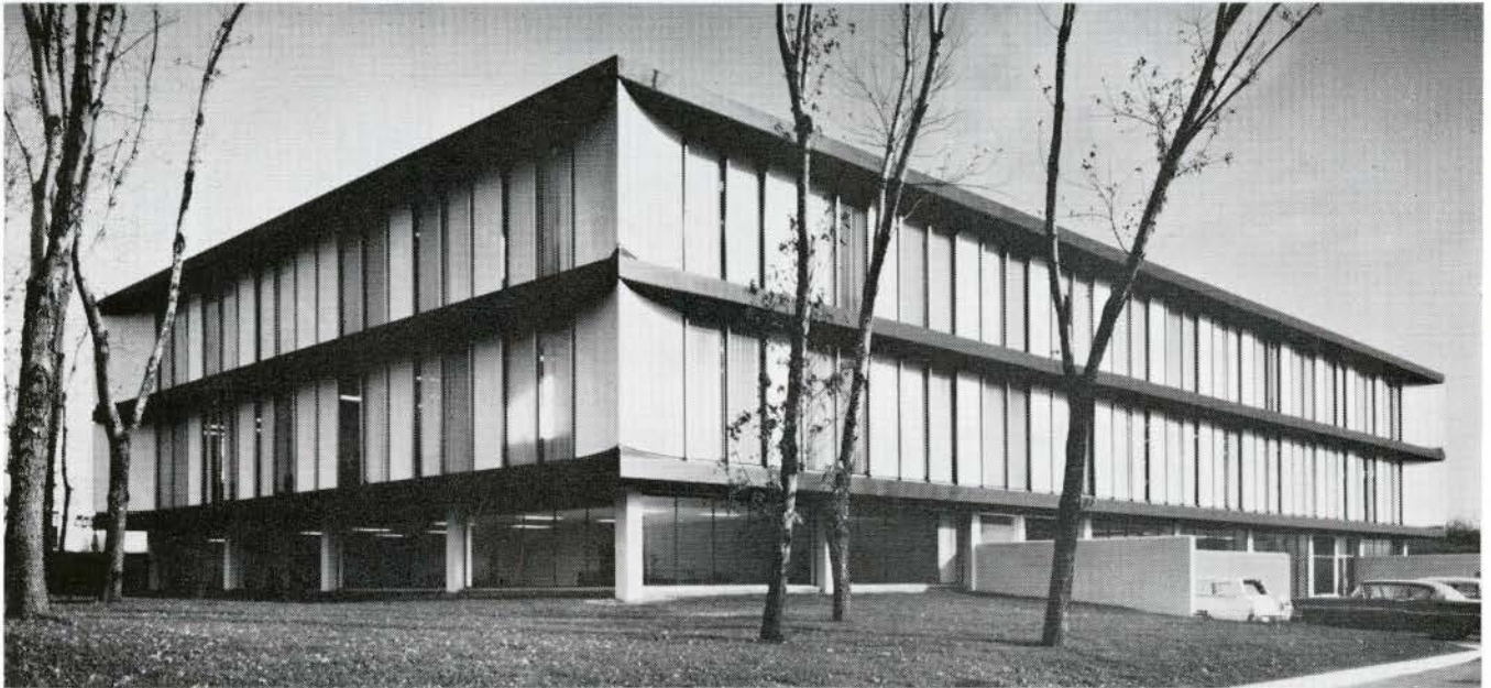
A. C. Nielsen Company of Canada Limited, Flemingdon Park, Don Mills, Ontario. Webb Zerata Menkés, Architects. General Contractors: Dell Construction Co. Limited.
