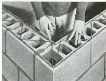
STRENGTH WITH FLEXIBILITY —this basic masonry wall requirement is met for sure (and economically!) when Dur-o-wal, above, is used with the ready-made, self-flexing Rapid Control Joint, below.
