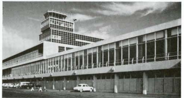
Twindow installation at Montreal International Airport, Dorval, P.Q.
