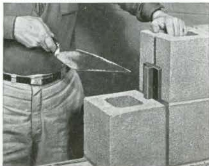
STRENGTH WITH FLEXIBILITY —this basic masonry wall requirement is met for sure (and economically!) when Dur-o-wal, above, is used with the ready-made, self-flexing Rapid Control Joint, below.
