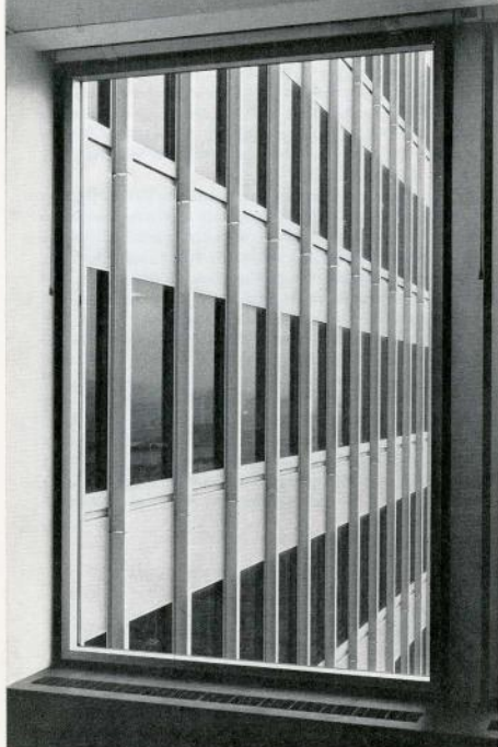
Interior and exterior detail of aluminum curtain wall, Place Ville Marie
