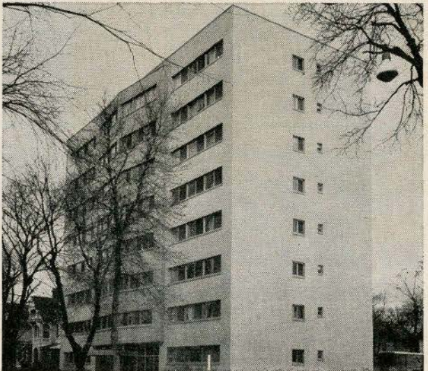
LINCOLN TOWERS APARTMENTS —General Contractor: Winnipeg Construction Company, Winnipeg Architect: Macleod and Reimer, Winnipeg
