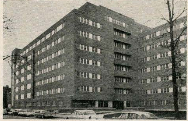
DEER LODGE HOSPITAL —General Contractor: Bird Construction Company Limited, Winnipeg Architect: Moody, Moore and Partners, Winnipeg
