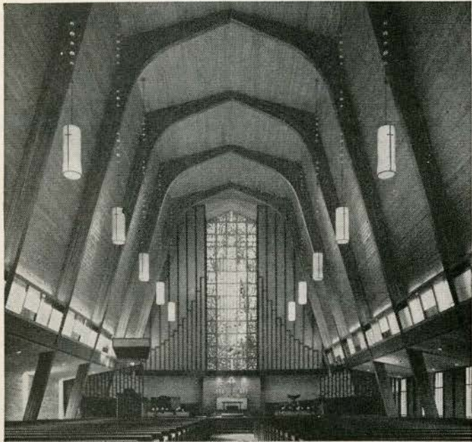
Massive laminated members supporting a planked ceiling uphold wood's strength and versatility. From pews to peak, wood's warmth is at work.
