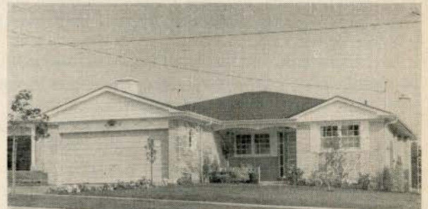
Shutters, scalloped friezes, panelling, and stone are used to soften and "sweeten" the house exterior. This is what the public appears to want
