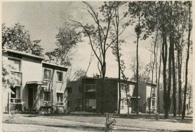
Quadruplex in Seignory Park. Architects: Affleck, Desbarats, Dimakopoulos, Lebensold, Michaud, Sise
