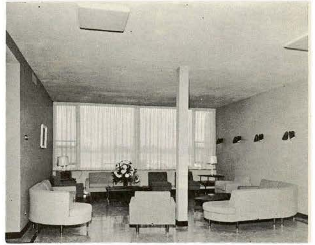
Above: Interior of the entrance lobby. Below: The patients sitting room.
