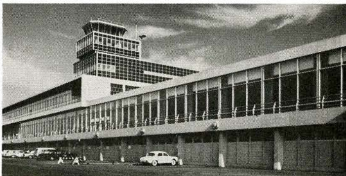
Twindow installation at Montreal International Airport, Dorval, P.Q. ARCHITECTS: Illsley, Templeton & Archibald, Larose & Larose, Associated Architects GENERAL CONTRACTOR: The Foundation Company of Canada Limited GLAZING CONTRACTOR: Canadian Pittsburgh Industries Limited
