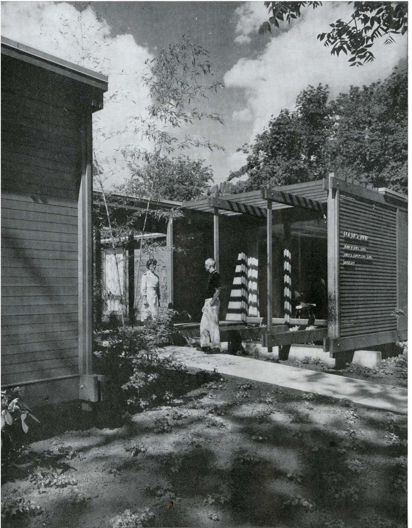
A unique dental clinic attests best to wood's natural adaptability and warmth. The simplicity of exposed beams and supports bolted together, the mixture of spaced and solid siding complementing one another—all present a friendly outside, promise a comfortable inside.
