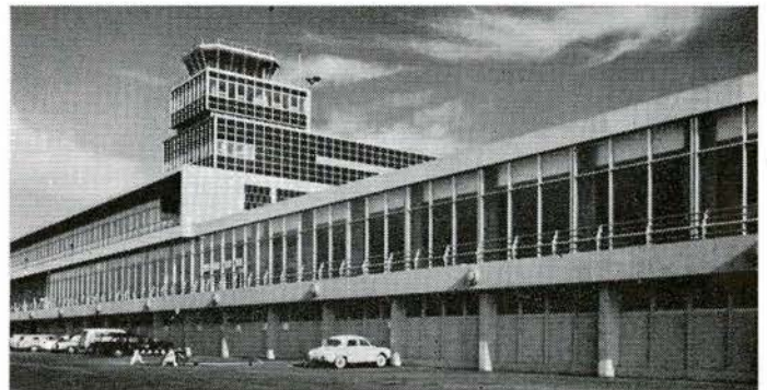
Twindow installation at Montreal International Airport, Dorval, P.Q. ARCHITECTS: Illsley, Templeton & Archibald, Larose & Larose, Associated Architects GENERAL CONTRACTOR: The Foundation Company of Canada Limited GLAZING CONTRACTOR: Canadian Pittsburgh Industries Limited
