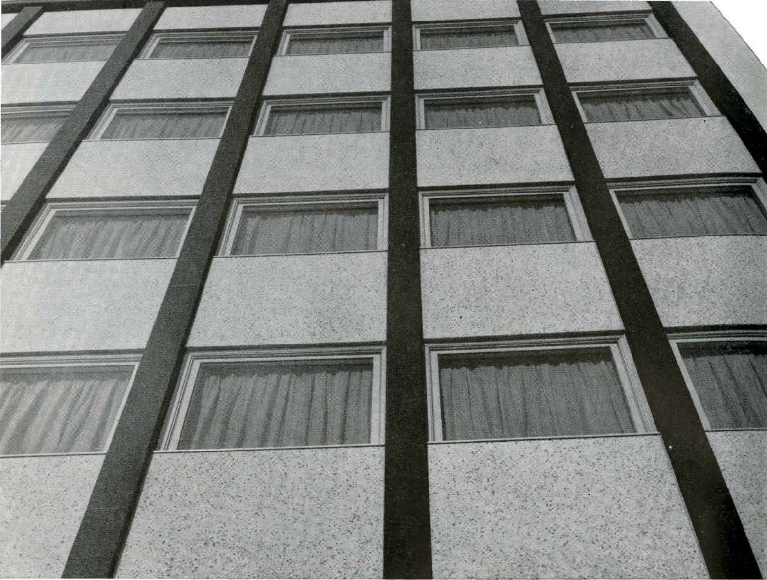
A Precast concrete panels with exposed aggregate add interest to this modern exterior.
