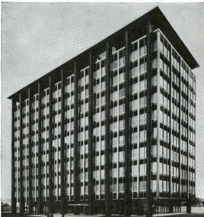
BUILDING: Union Carbide Canada Limited, Toronto, Ontario ARCHITECT: Shore and Moffatt, Toronto GENERAL CONTRACTOR: Anglin-Norcross Ontario Limited
