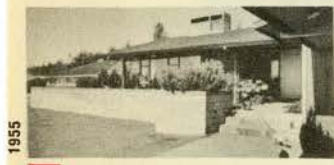
9 Taylor Residence 605 King George Way. Architects: J. Blair MacDonald & Clyde Rowett
