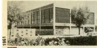
5 BC Telephone Exchange Tenth Ave. at Tolmie. Architects: McCarter Nairn and Partners
