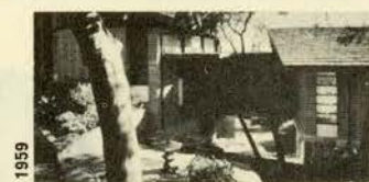
16 R. A. Chillcott Residence 3990 Bayridge. Architects: Duncan McNab and Associates
