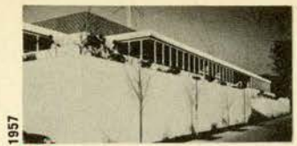
3 Radio Station CKWX* 1275 Burrard Street. Architects: Thompson, Berwick and Pratt
