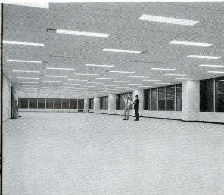
Steel permits longer spans for a given beam dimension than is practical with other materials.
