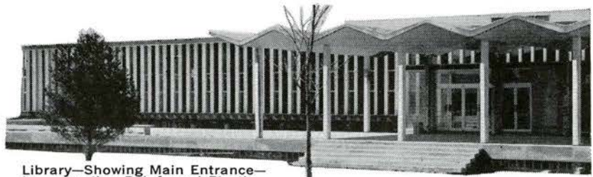
Library—Showing Main Entrance— Incorporating Reinforced Plastic Fins and Panels.
