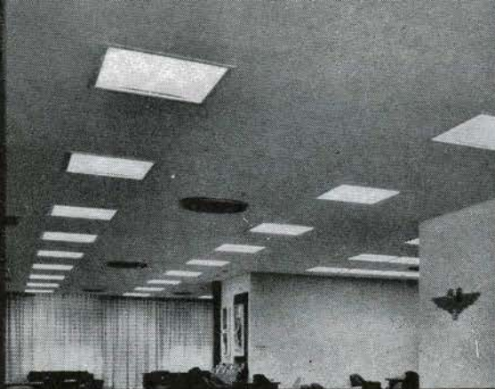
Airways Sales Office . . . Recessed Luminaires
