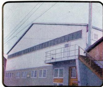
Fish Packing Plant: B.C. Packers Ltd., Vancouver, B.C. Building Designer: Owner Aluminum Fabricator: Nesco Aluminum Ltd.
