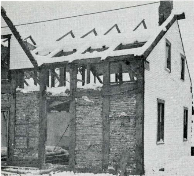
FIG 8 Wood frame and brickwork construction.
