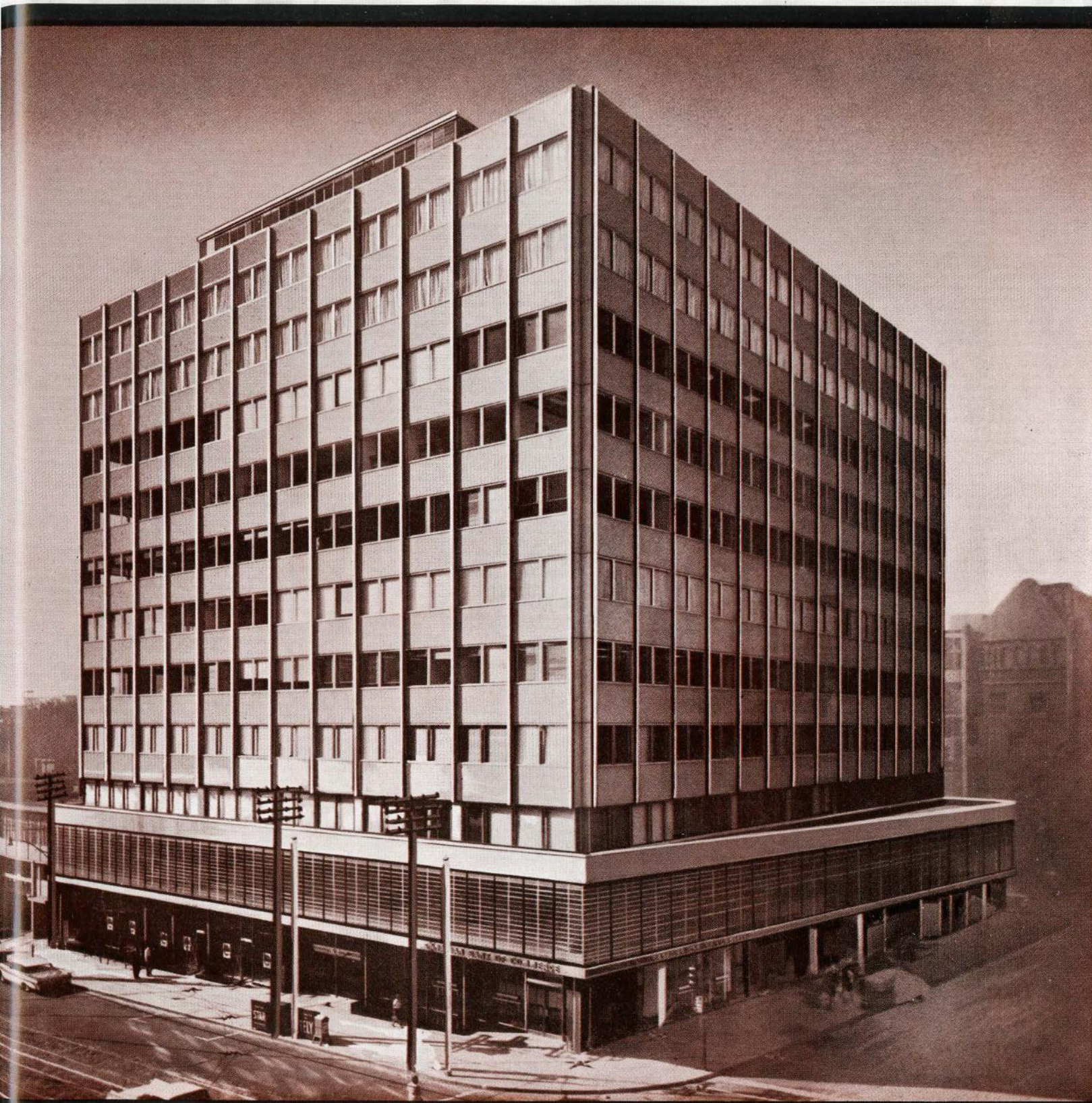
• MO-SAI CURTAIN WALL FOR OFFICE BUILDING, 790 BAY ST., TORONTO. ARCHITECTS: PETER DICKINSON & ASSOCIATES
