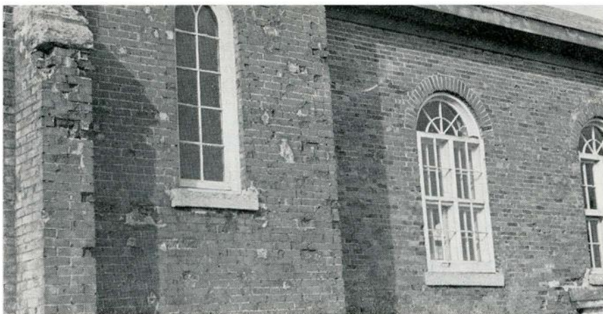
FIG 11 Spalled bricks and damaged buttress of church at Dickinson's Landing.
