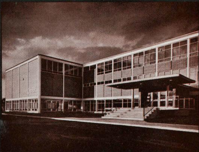
• EXPOSED STRUCTURAL FRAMEWORK WILLOWDALE JUNIOR HIGH SCHOOL, WILLOWDALE, ONT. ARCHITECTS: PAGE AND STEELE. ENGINEERS: M. S. YOLLES AND ASSOCIATES
