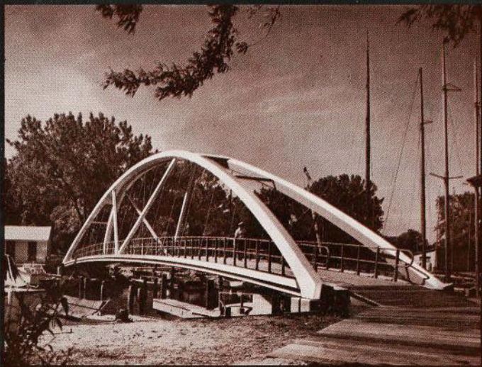
• 160' SPAN BOW-STRING BRIDGE FOR ROYAL CANADIAN YACHT CLUB, TORONTO ENGINEERS: LAURENCE CAZALY
