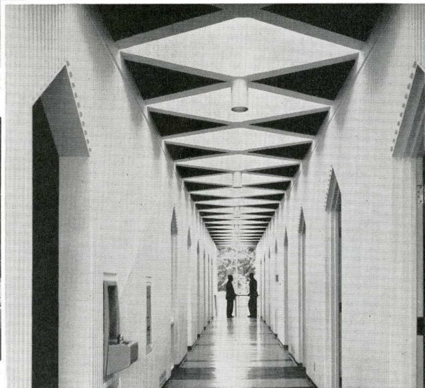
X-SHAPED BEAMS create diamond-shaped skylights in the central corridor where precast roof segments meet.
