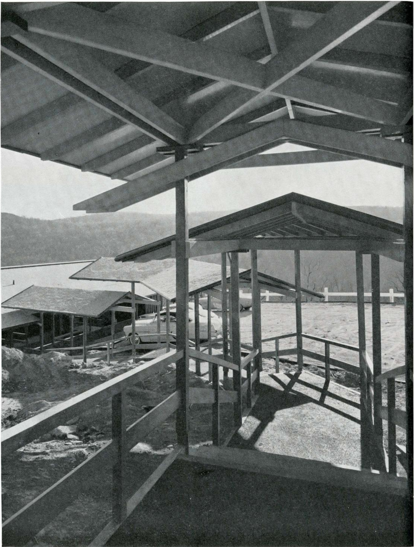
Chosen for its workability and ability to blend with the beauty of the landscape, straight grain wood is utilized in exposed framing throughout the Motel on the Mountain.
