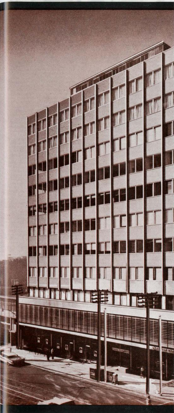
• MO-SAI CURTAIN WALL FOR
