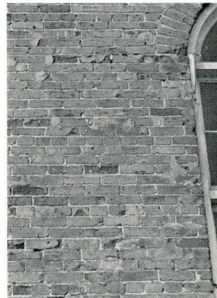
FIG 11 Spalled bricks and damaged buttress of church at Dickinson's Landing.
