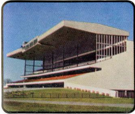
Race Track Grandstand & Clubhouse: Ontario Jockey Club Ltd., Malton, Ont. Architect: Earle C. Morgan Aluminum Fabricator & Erector: Robertson-Irwin Ltd.
