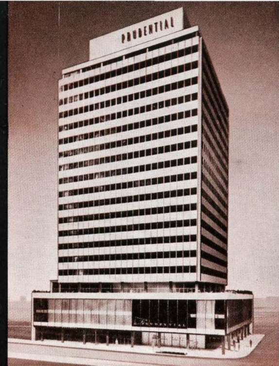
• MO-SAI CURTAIN WALL PRUDENTIAL INSURANCE CO. OF AMERICA, TORONTO ARCH. PAGE & STEEL AND PETER DICKINSON & ASSOC.
