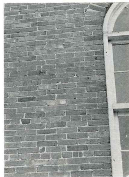
FIG 10 East and west walls of the church at Dickinson's Landing (erected 1863), the east wall (bottom) showing much greater effects of weathering.
