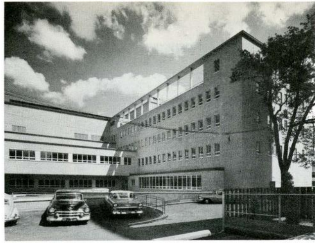
West elevation: courtyard and small parking area
