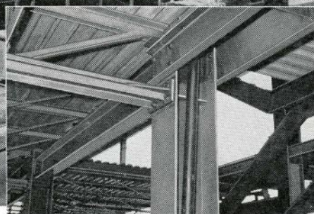
BESIDES PROVIDING continuous shallow depth floor girders, twin channels placed on opposite flanges of the columns allow more efficient positioning of vertical pipe runs.
