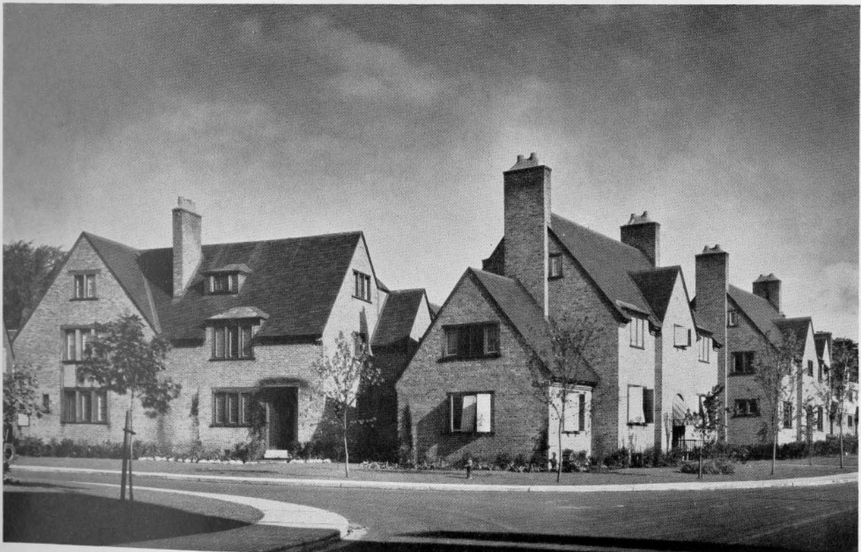
CORNER OF BARAT PLACE AND DE CASSON CRESCENT, WESTMOUNT Shorey & Ritchie, Architects
