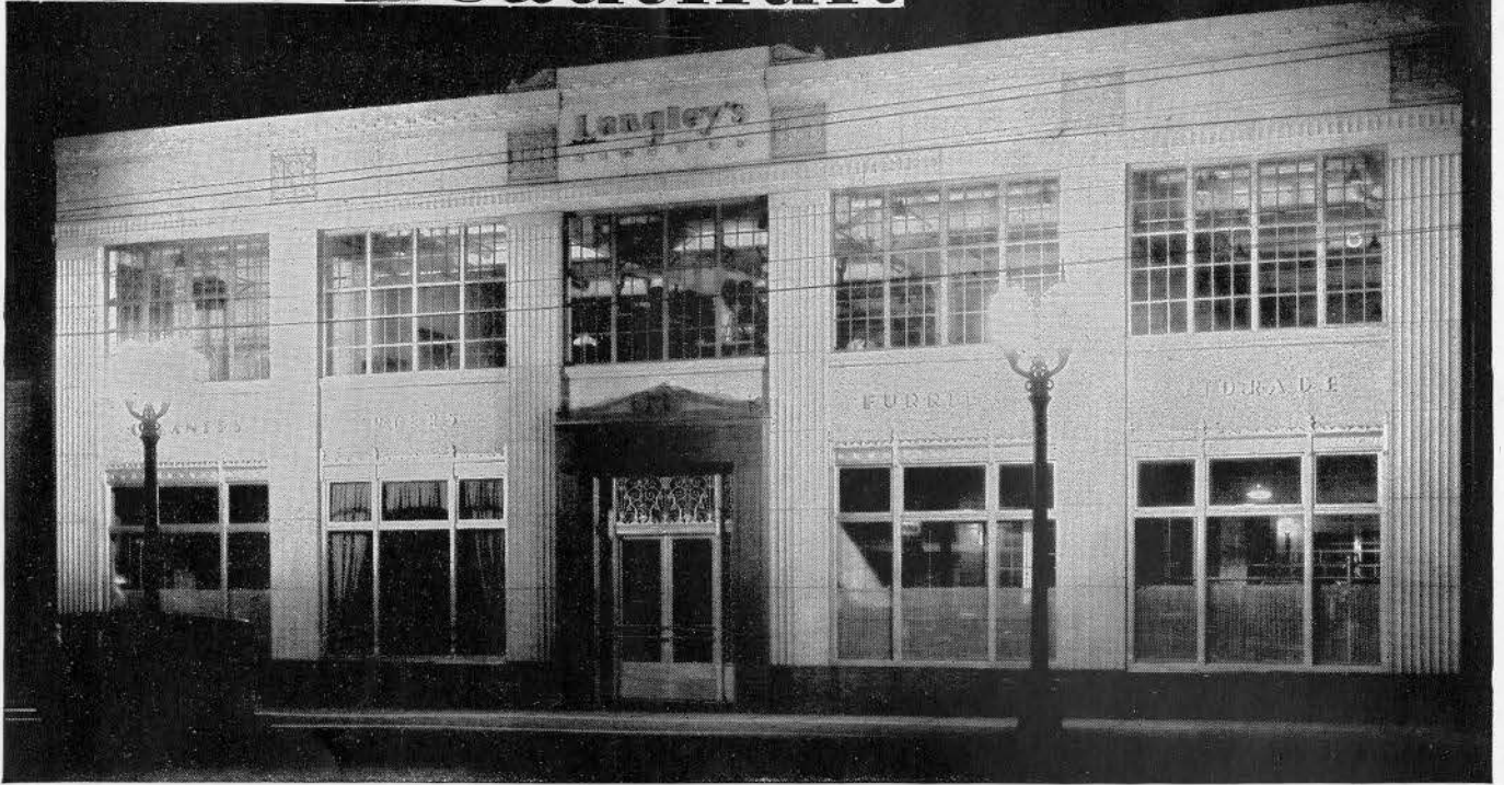
The new Langley Building, Hamilton, is lighted by two Westinghouse Duolux standards, each lighting unit being equipped with two 1,000 watt lamps for floodlighting the building and two 200 watt lamps for lighting the sidewalk.
