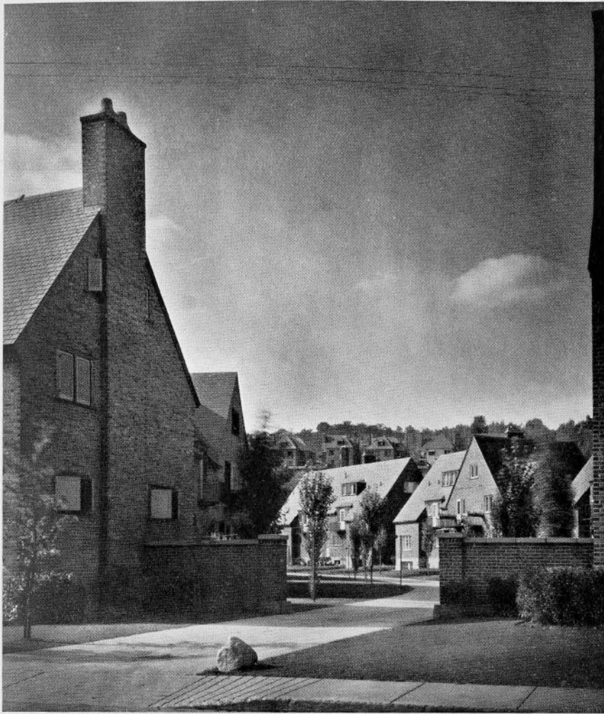
ENTRANCE TO LANE AND GARAGES AT REAR OF HOUSES FACING HOLTON AVE. AND DE CASSON CRESCENT, WESTMOUNT
