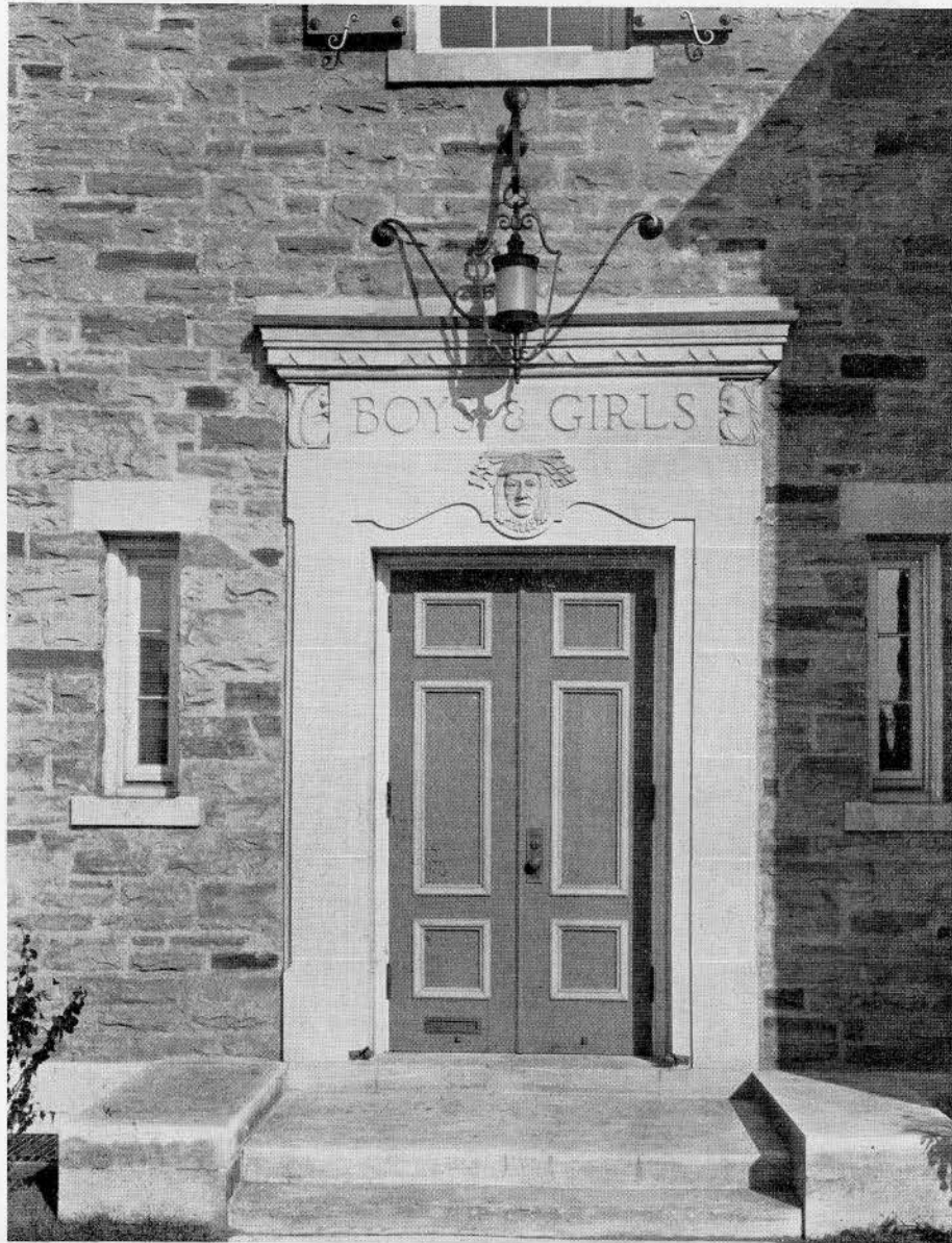
DETAIL, BOYS' AND GIRLS' ENTRANCE, RUNNYMEDE BRANCH LIBRARY John M. Lyle, R.C.A., F.R.A.I.C., Architect
