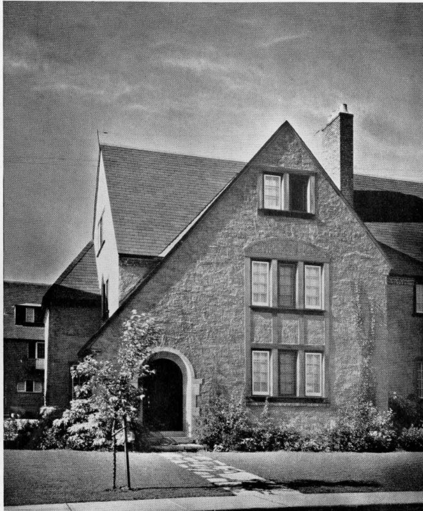
SEMI-DETACHED RESIDENCE ON DE CASSON CRESCENT, WESTMOUNT
