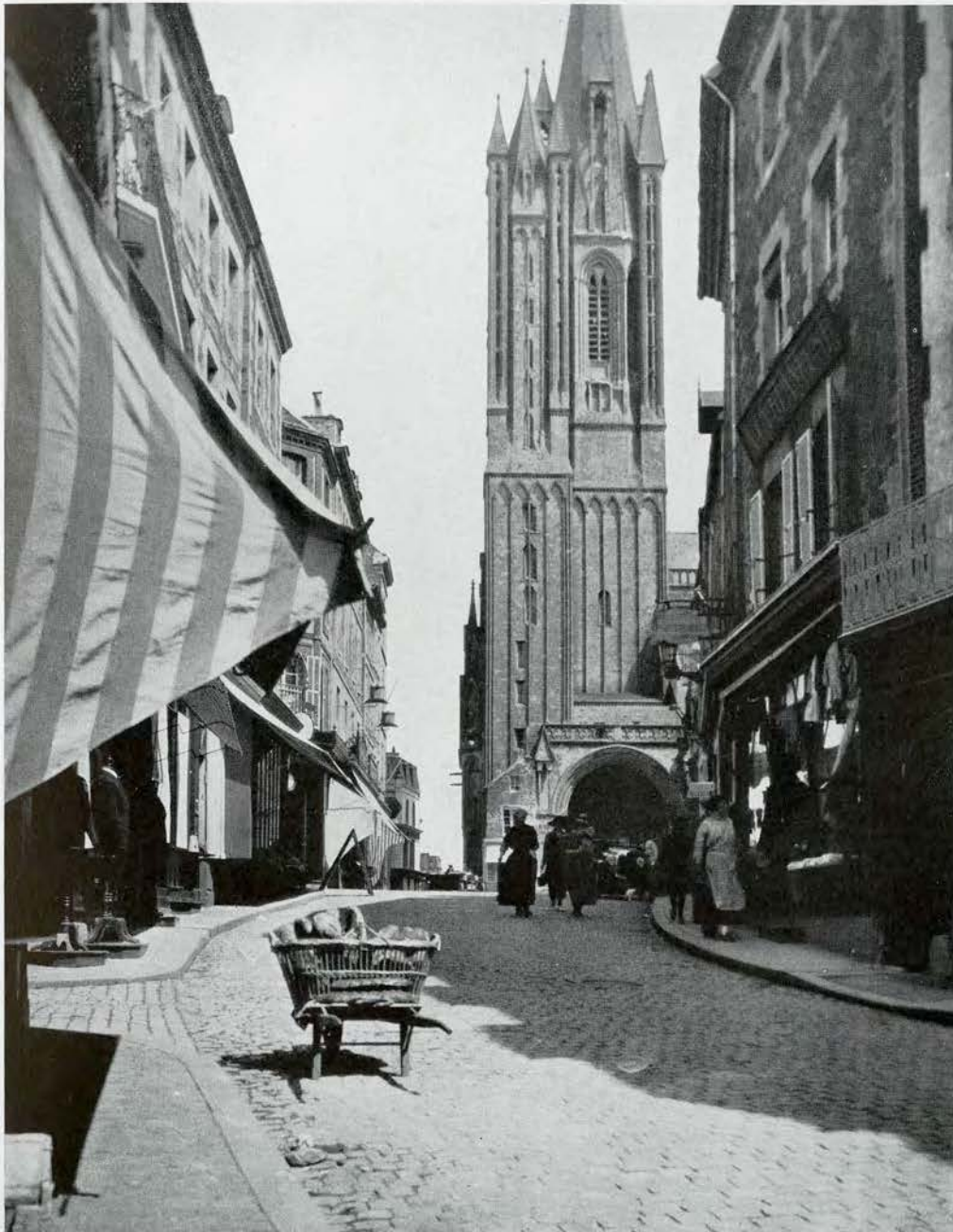
SOUTH TOWER, COUTANCES CATHEDRAL, FRANCE
