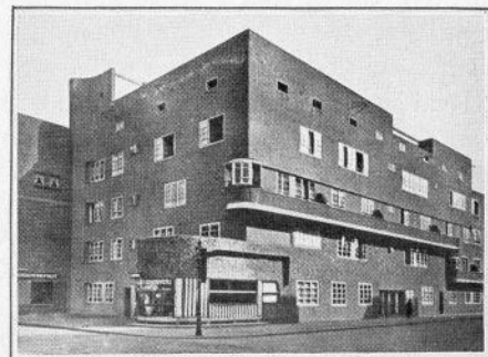
Supposing the haphazard placing of windows is demanded by the plan, and that the corner shop is commercially efficient, why thin the wall of the storey above the balcony?
