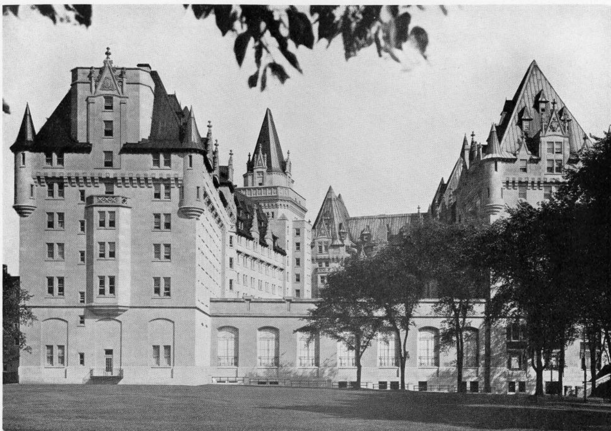
REAR VIEW OF THE NEW CHATEAU LAURIER
