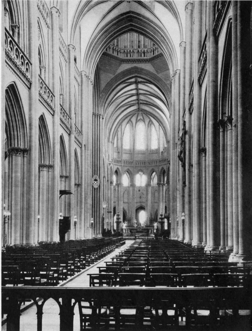
NAVE, COUTANCES CATHEDRAL, FRANCE
