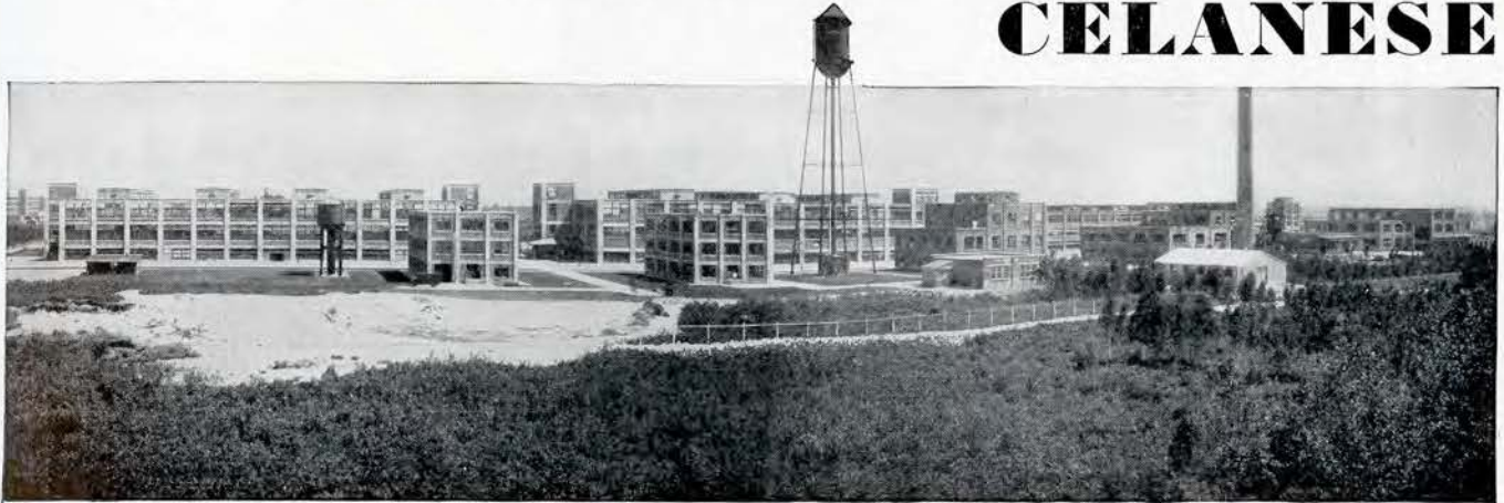
CANADIAN CELANESE, LIMITED, Drummondville, P. Q. 99,247 sq. ft. of Barrett Specification Roofs protect this mammoth plant—one of the finest in the Dominion. Architects and engineers: Canadian Celanese, Limited.
