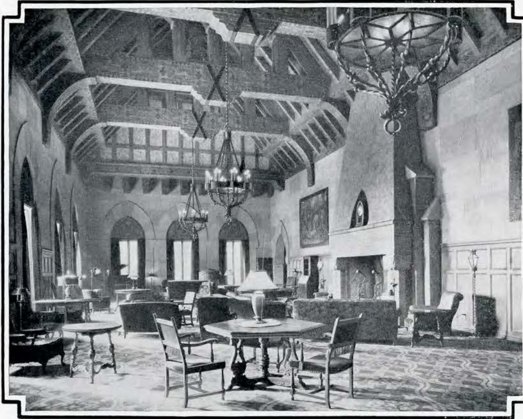
Trusses of reinforced concrete, richly decorated, provide a picturesque and traditional beauty in the lounge of the Pacific Coast Club, Los Angeles.
