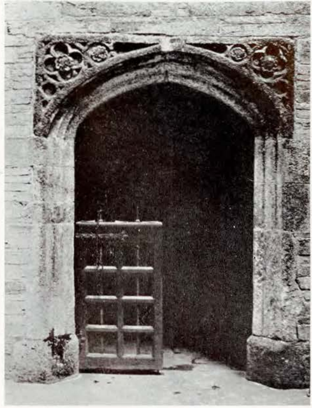
ENTRANCE TO PORCH
