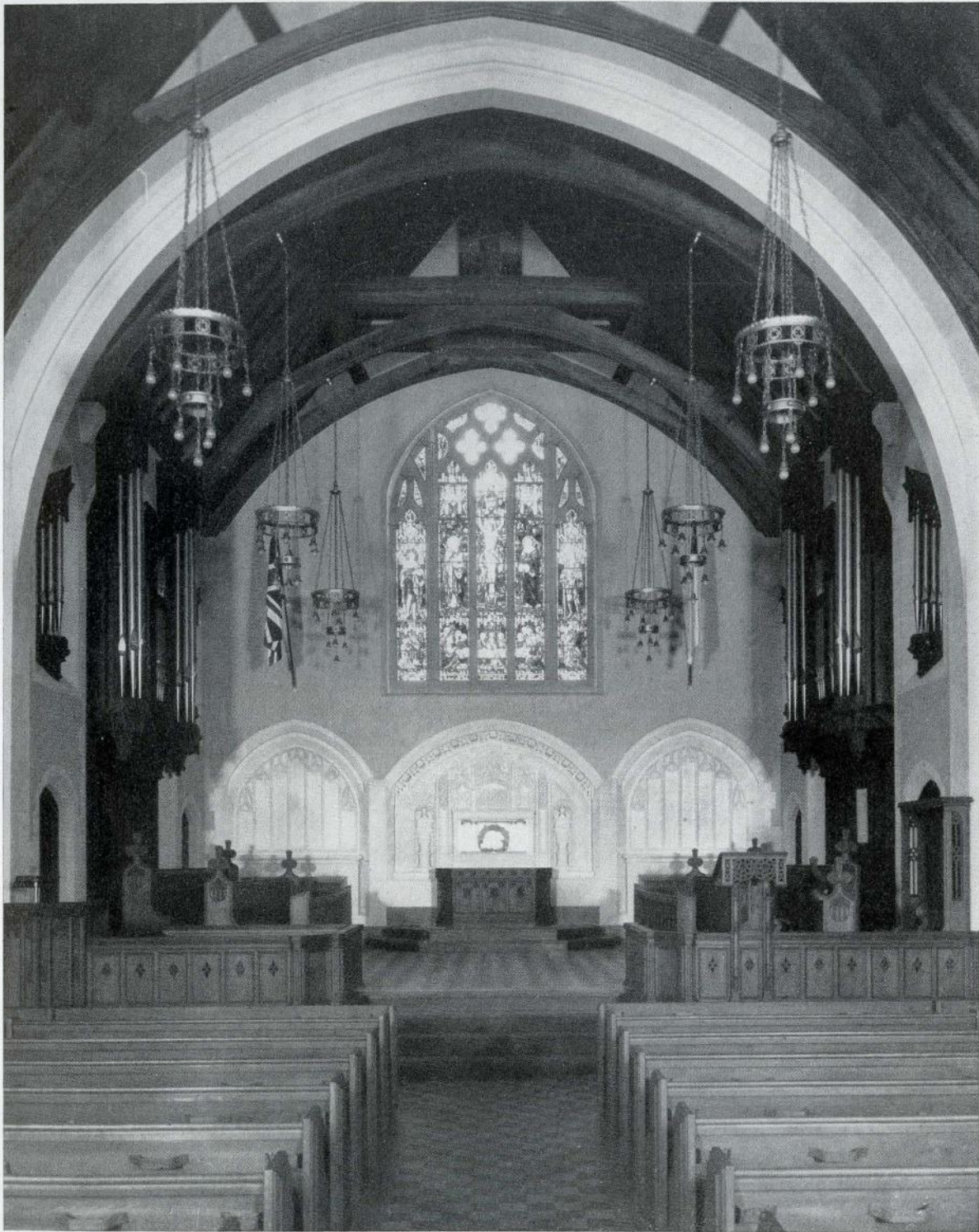
INTERIOR, LOOKING TOWARDS CHANCEL, CANADIAN MEMORIAL CHAPEL, VANCOUVER, B.C. Twizell & Twizell, Architects
