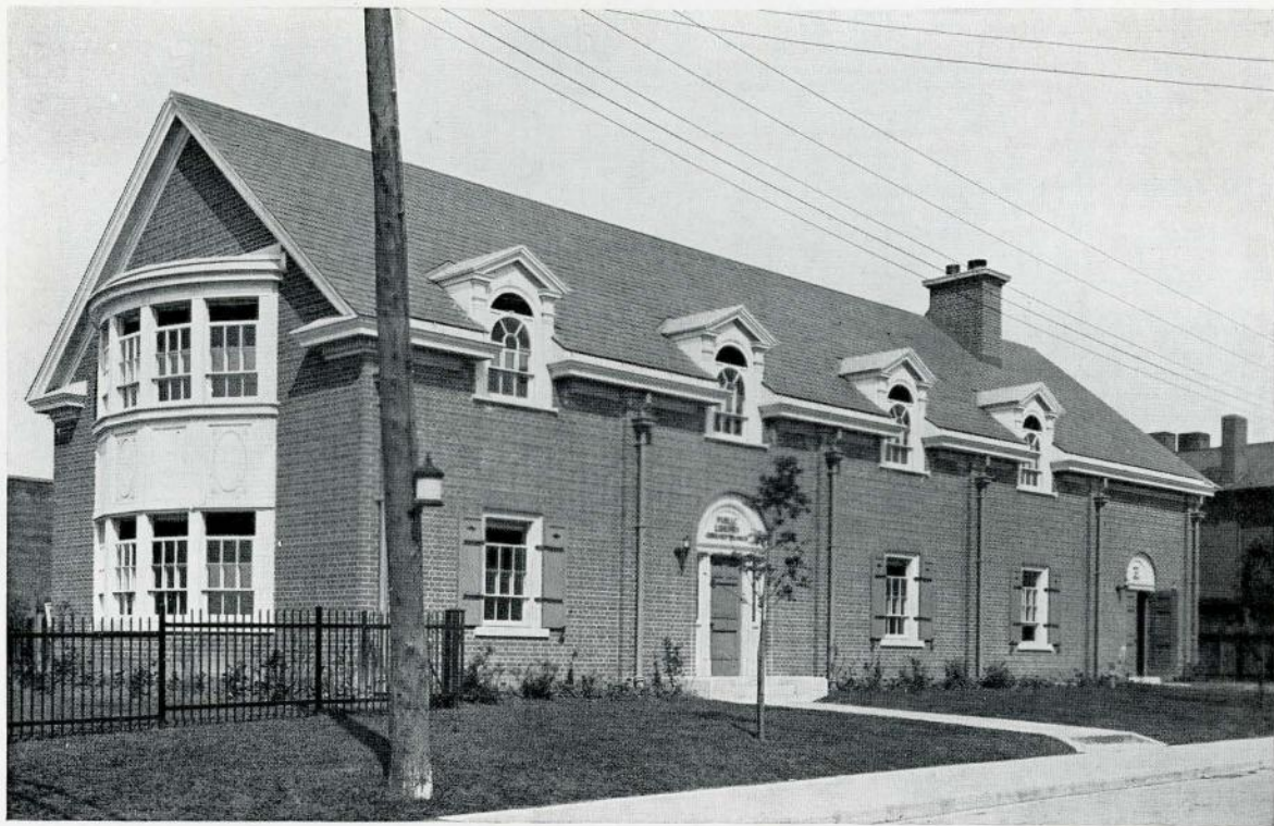
GERRARD BRANCH, TORONTO PUBLIC LIBRARY Shepard & Calvin Architects
