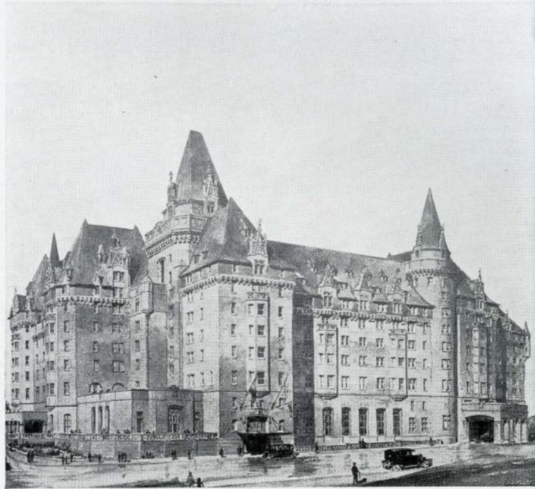
EXTENSION TO CHATEAU LAURIER, OTTAWA John S. Archibald, F.R.S.A., Architect Foundation Company, Montreal, General Contractors
