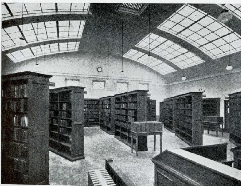
INTERIOR OF LENDING LIBRARY. NEW PUBLIC LIBRARY, WATFORD, ENGLAND
