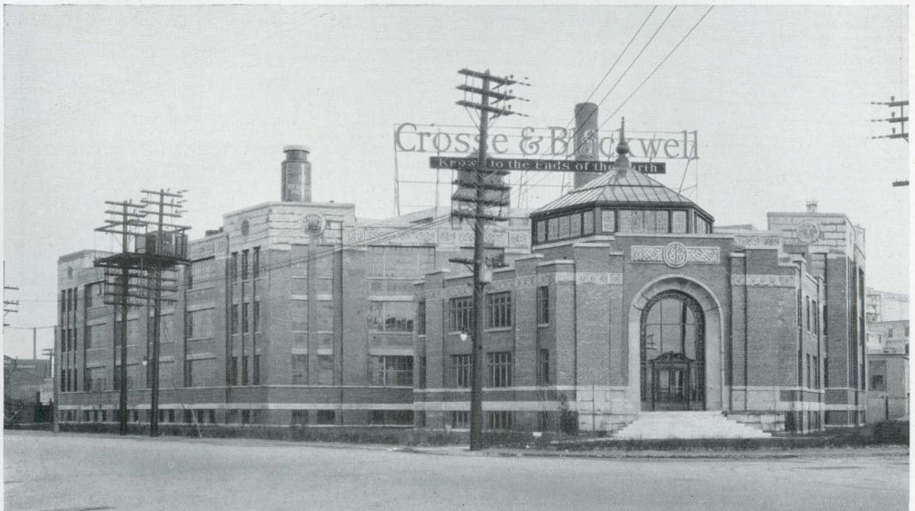
HONOURABLE MENTION—INDUSTRIAL BUILDINGS. CROSSE & BLACKWELL BUILDING, TORONTO Chapman & Oxley, Architects
