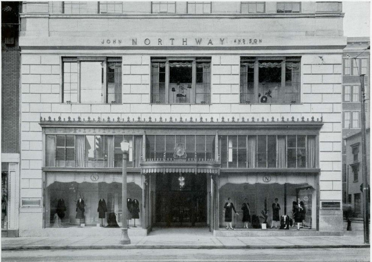
HONOURABLE MENTION—SHOP FRONTS. NORTHWAY STORE, TORONTO Horwood & White, Architects
