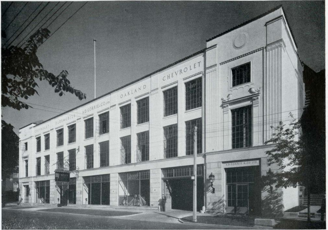
FIRST AWARD—COMMERCIAL GARAGES. A. D. GORRIE GARAGE, TORONTO Murray Brown, Architect
