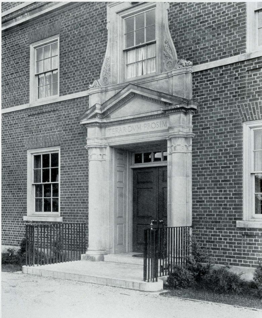
SECOND AWARD—DETAILS, DOMESTIC. FRONT ENTRANCE, LOWER SCHOOL OF RIDLEY COLLEGE, ST. CATHARINES, ONTARIO Marani, Lawson & Paisley, Architects
