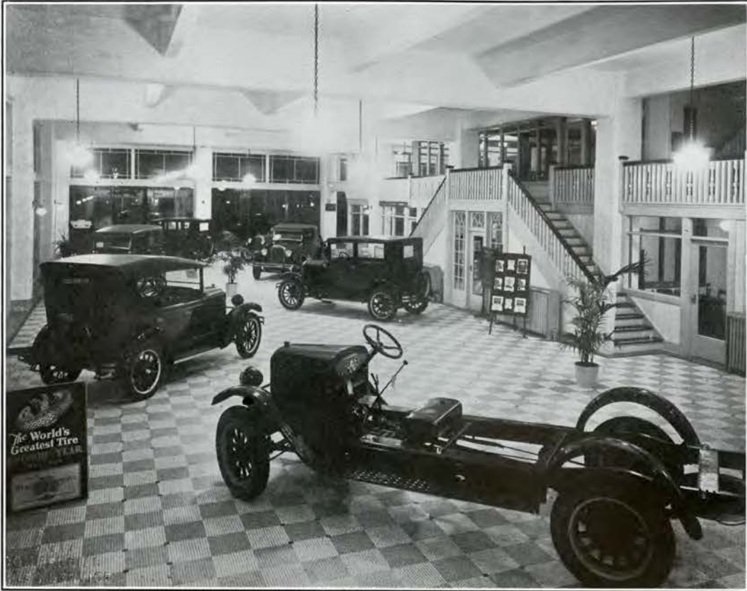
A perfect job of showroom illumination in Vancouver with Westinghouse Fixtures
