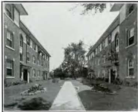
WALPAMUR was used in the BURINN APARTMENTS off Broadway Avenue, Toronto. Built by W. Pidgeon.
