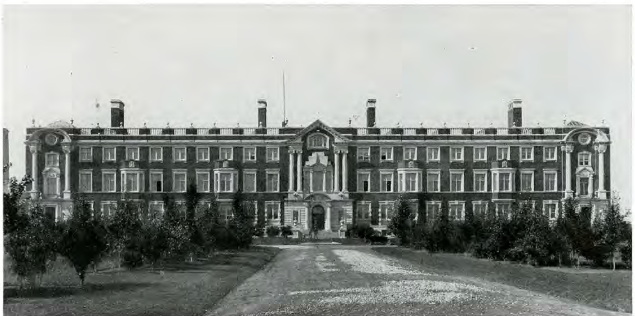
ARTS BUILDING, FRONT VIEW, UNIVERSITY OF ALBERTA Nobbs & Hyde, Architects
