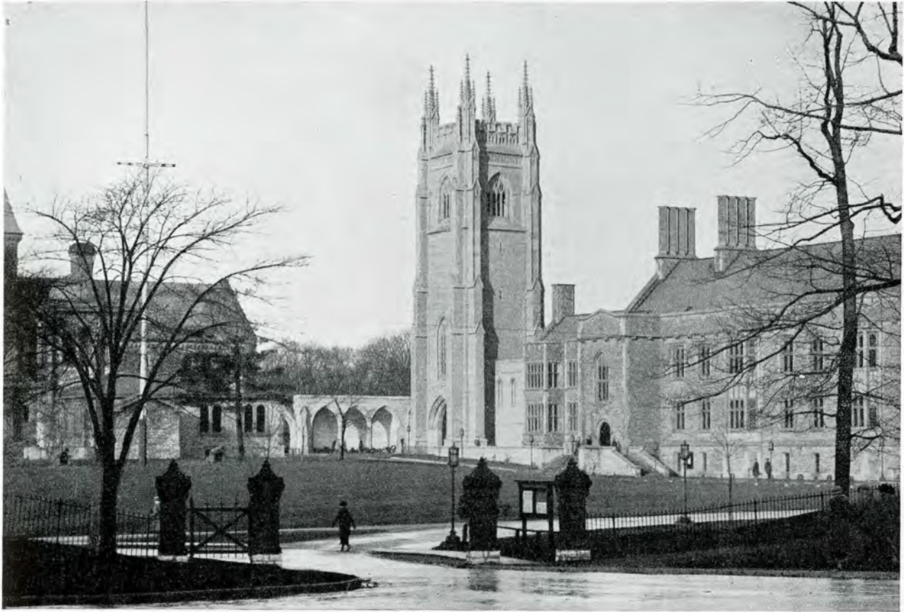
WAR MEMORIAL TOWER, FROM SOUTH-EAST—UNIVERSITY OF TORONTO Sproatt and Rolph, Architects
