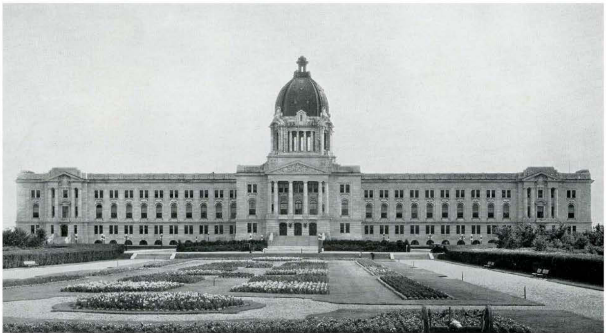
FRONT ELEVATION (PHOTOGRAPH), SASKATCHEWAN LEGISLATIVE BUILDINGS Edward & W. S. Maxwell, Architects
