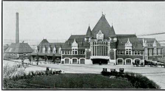
Canadian Pacific Railroad Terminal in Quebec Waterproofed with No. 232 "R.I.W."
