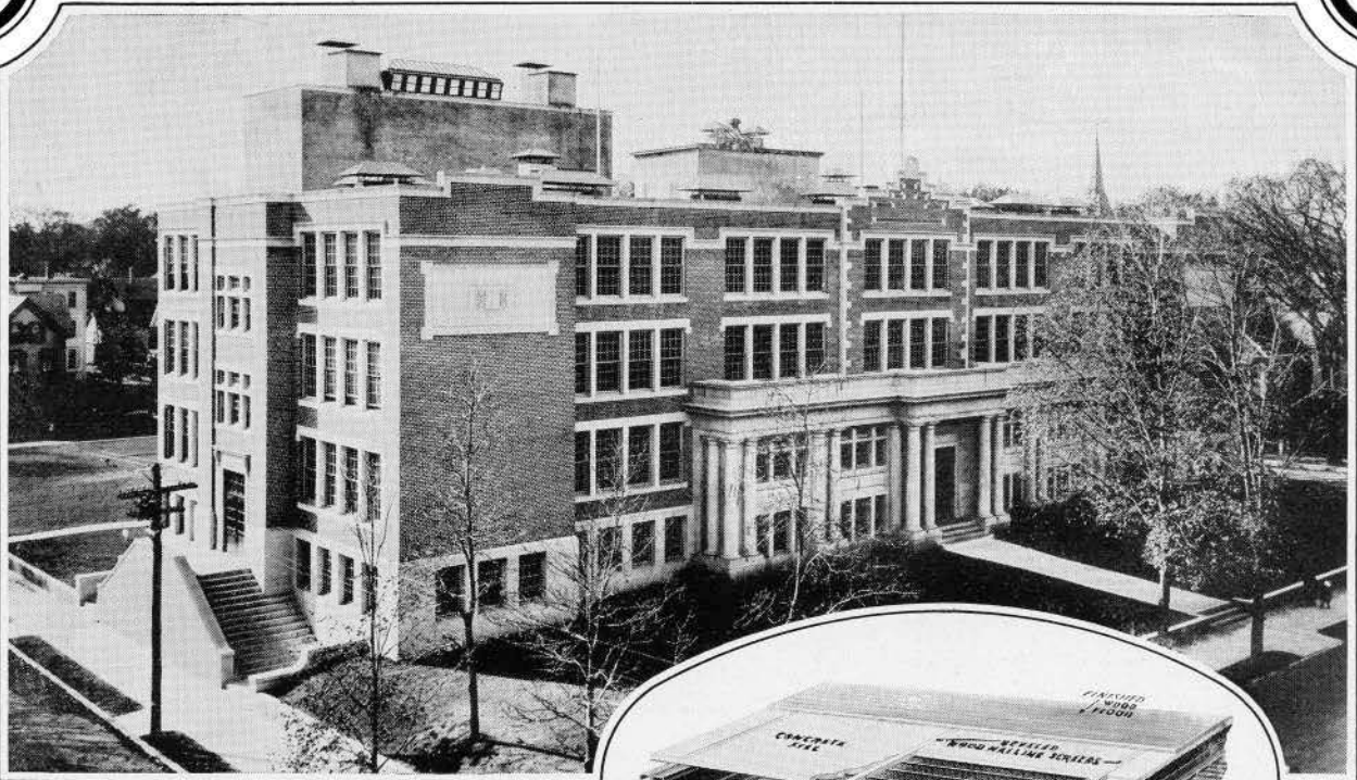
TRUSCON STEEL JOISTS ARE USED THROUGHOUT IN THIS HIGH SCHOOL
