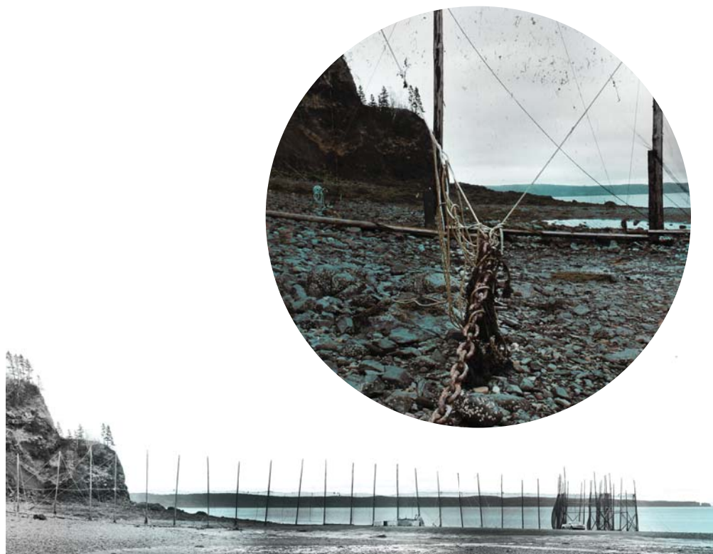
Below: Fishing weir at Partridge Island, shown at low tide, with Cape Split in the background. These vernacular structures serve as a precedent for the structure of the proposed boat bridge. Right: Detail of the fishing weir ground connection.
