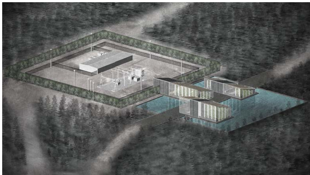
Isometric view of the upper reservoir and community greenhouse at the high water level, in relation to the existing substation.
