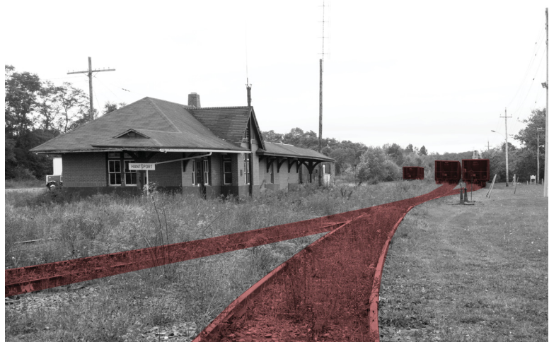
Figure 31: Abandoned railroad line.
