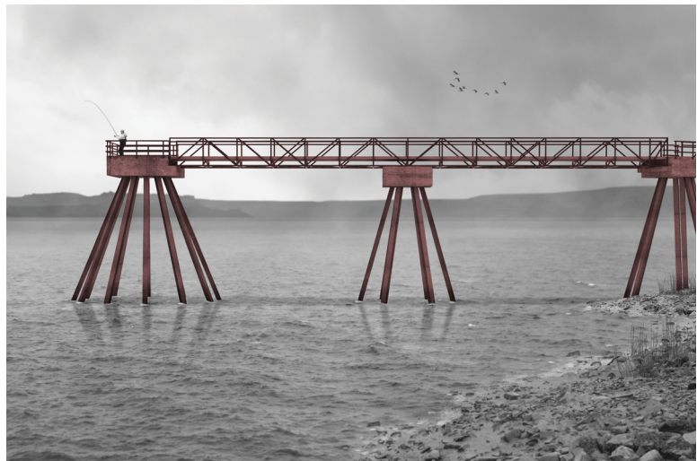
Figure 62: The gypsum pier tidal walk.
