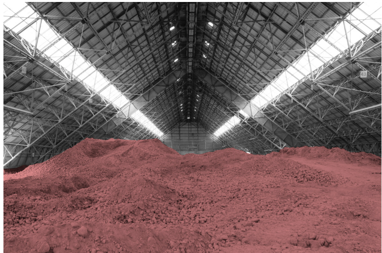
Figure 32: Interior of gypsum storage shed, gypsum piled high.
