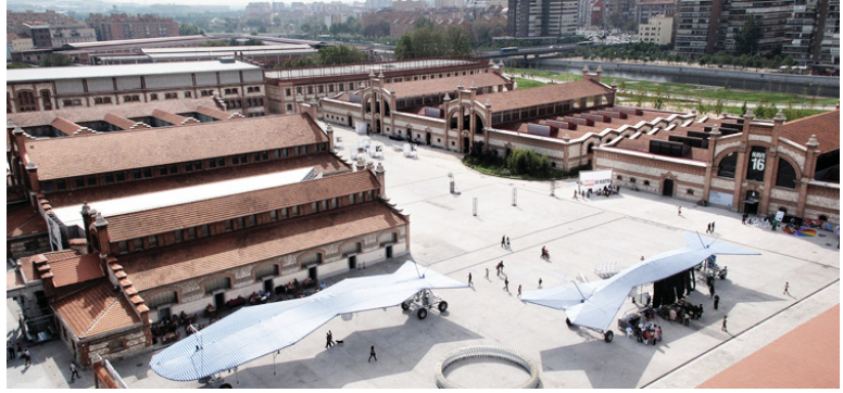
Figure 23: An aerial view of the Matadero plaza and surrounding buildings; from Architectours in Madrid Río y Matadero Madrid.
