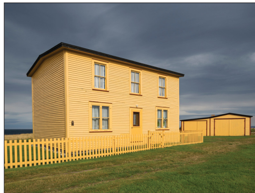
TYPICAL 1900'S BUILDING WITH A SIMPLE PAINT SCHEME AND OUTBUILDINGS (RESTORED)
