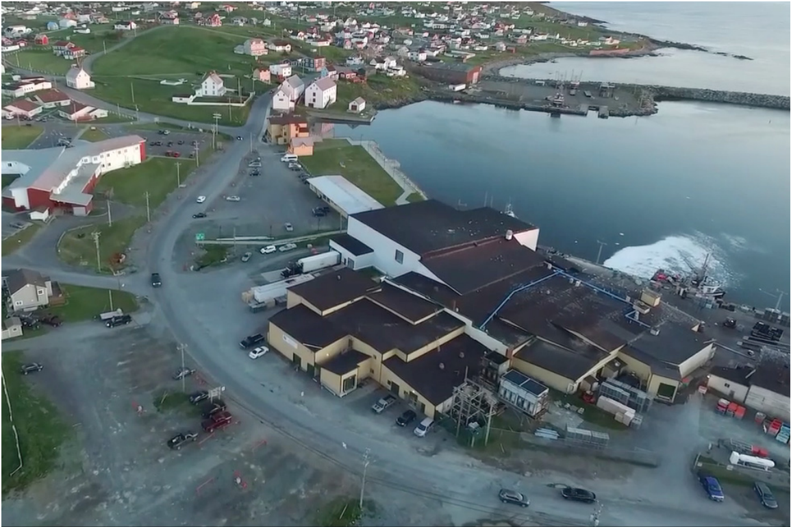
Fig.65 Exterior of the Fish Plant in Bonavista depicting the epitome of a practical, functional response to a problem of needing additional space, again and again over the years. Source: Cahill, Kevin. 2016.
