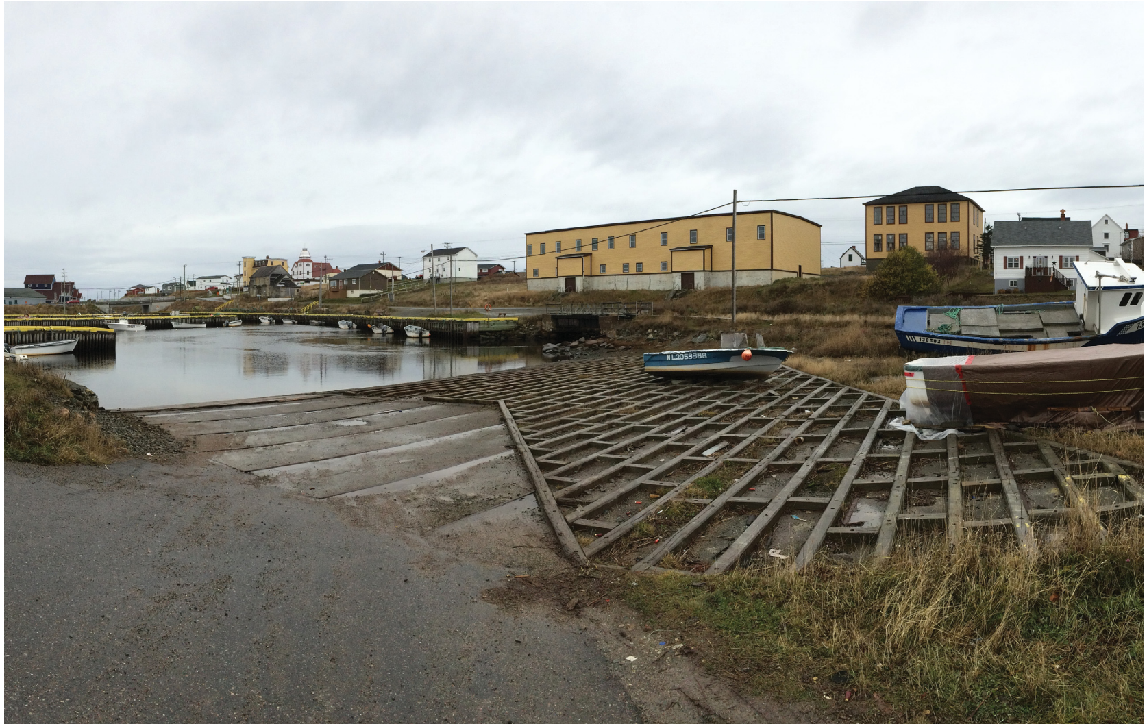
Fig.88 The two schools and the site, with frontage on the only protected harbour in Bonavista.
