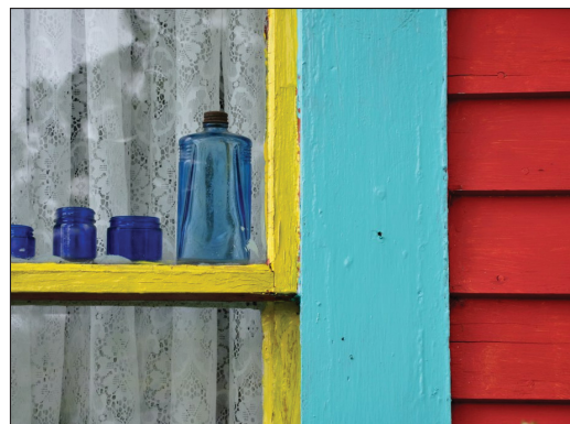
OVERALL DISSONANCE. A DETAIL THAT ILLUSTRATES SEVERAL CONDITIONS: PAINT PEELING, BUILDUP, AND COLOR CHANGE (LEFT-RIGHT).
