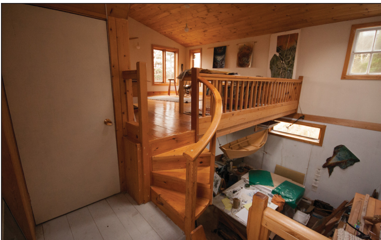
Fig.13 The upper floor entry from the old house into the artist studio addition.
