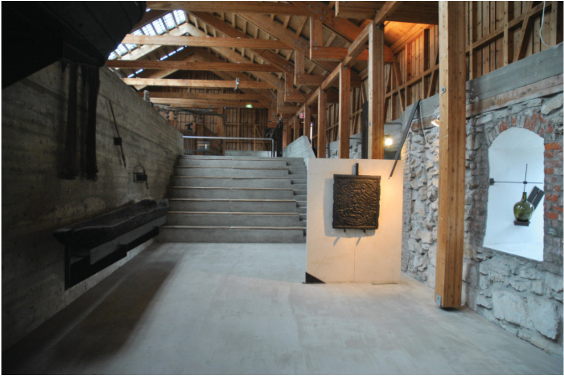
Fig.62 Interior of the Hedmark Museum in Hamar, Norway, showing the clear distinction between old and new structure, carefully touching the partially restored existing building. The new concrete benches and elements are get close to the old, but accentuate them rather than absorb or out-due them. Source: Umanskay, 2014.
