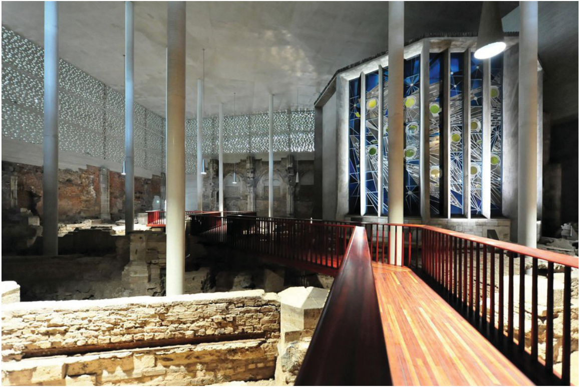
Fig.58 Interior of the Kolumba Museum in Cologne, Germany, which utilizes a very similar approach to Raphael Moneo's National Museum of Roman Art in Mérida, Spain. At its lower levels, the new structure rises out of the untouched ruins. Unlike Moneo, Zumthor uses slender juxtaposing columns rather than mimicking the arches. Source: Vazquez, 2010.
