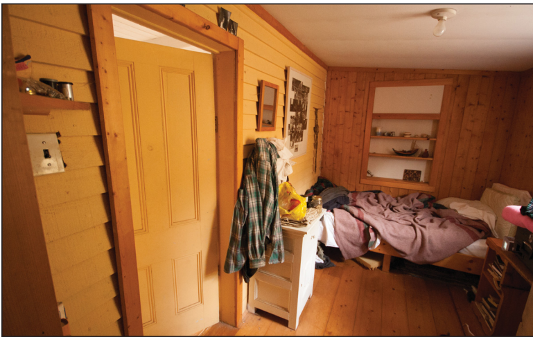
Fig.12 The rear addition interior features a bedroom and bathroom with the original exterior siding retained.
