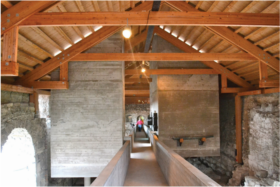
Fig.64 Interior of the Hedmark Museum in Hamar, Norway, showing the clear distinction between old and new structure, floating above the partially restored existing building. The wood roof and columns rest carefully on the existing and call attention to it. Circulation is controlled with the new elements to encourage a new way of moving around the building horizontally and vertically. Source: Umanskay, 2014.
