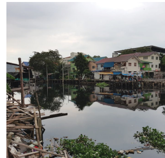
CONCRETE FLOOD WALLS ALONG CANAL
