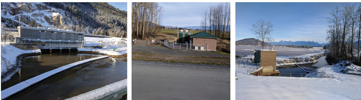
Barrowtown Pump Station (left), Collinson Pump Station (center), McGillivray Pump Station (right).
