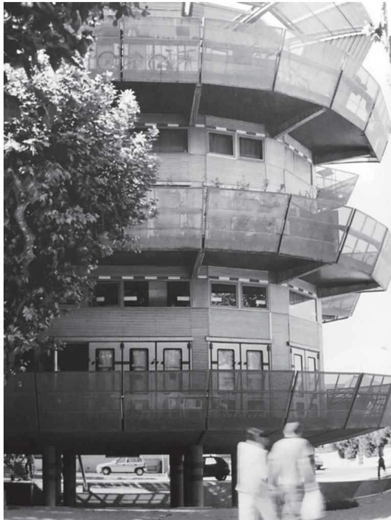
Figure 27 + 28. Georg Fessy, NEMAUSUS ; from Ramias Steinemann, "Global Housing Projects: 25 Buildings Since 1980."
