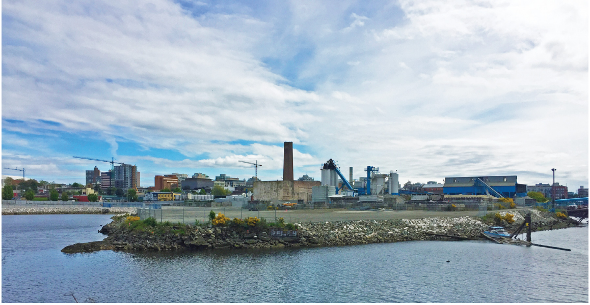
Figure 10: View looking south at The Powerhouse
