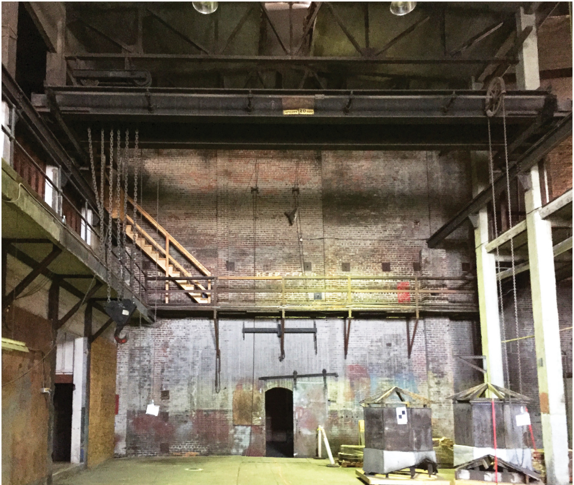
Figure 11: Large open interior space inside The Powerhouse
