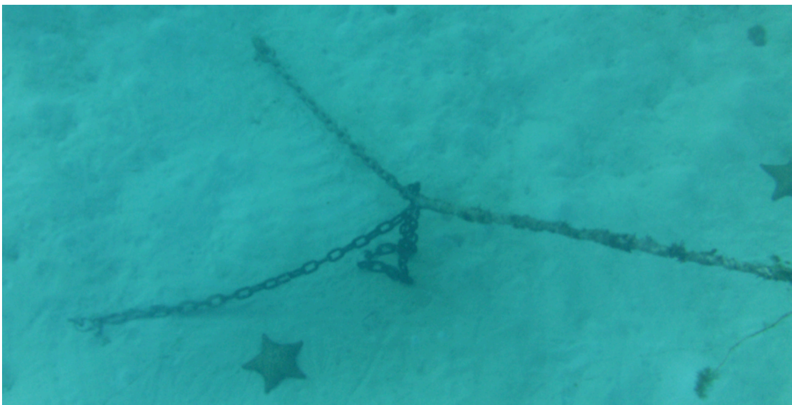
Figure 26. Image of manta and pin anchor with two pins, TCMP (Reed, 2016).
