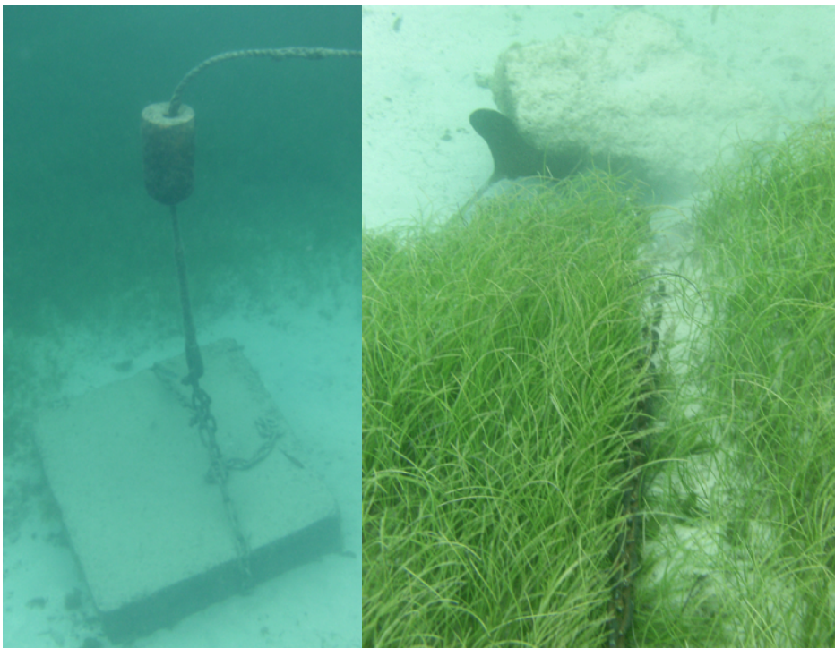
Figure 33. Image (left) showing concrete block anchor with chain and float that is preventing scouring of the surrounding seabed, TCMP (Reed, 2016).
