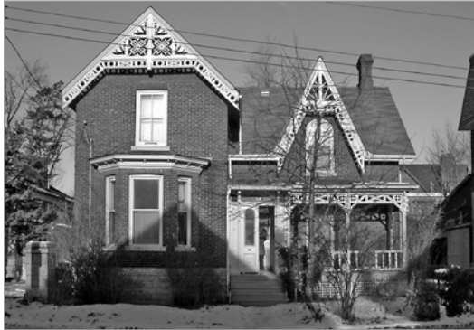
FIG. 44. "THE ONTARIO COTTAGE" LEGACY, 69 LOWER UNION ST., KINGSTON. | JENNIFER MCKENDRY.
