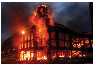
Destruction of union point building (Independent 2014)
