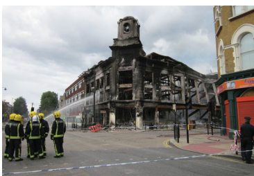
Destruction of union point building (Stanton 2011)
