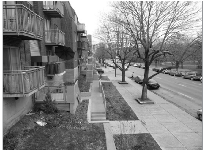
FIG. 12. BUILDINGS WITH GRASSED EMBANKMENTS, SUPPORT WALLS, AND STAIRS ON SAINT-JACQUES STREET. | MAUDE GILLES, 2015.
