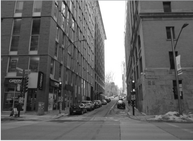
FIG. 27. ADAPTATION OF BUILDINGS TO THE TOPOGRAPHY BY WAY OF A PEDESTAL. | MAUDE GILLES, 2015.
