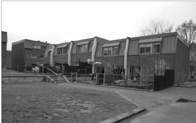
FIG. 13. REINTERPRETATION OF THE ROW-HOUSE TYPOLOGY AND PRESERVATION OF THE LINK TO THE LOT AND FRONT AND REAR YARDS. | MAUDE GILLES, 2015.
