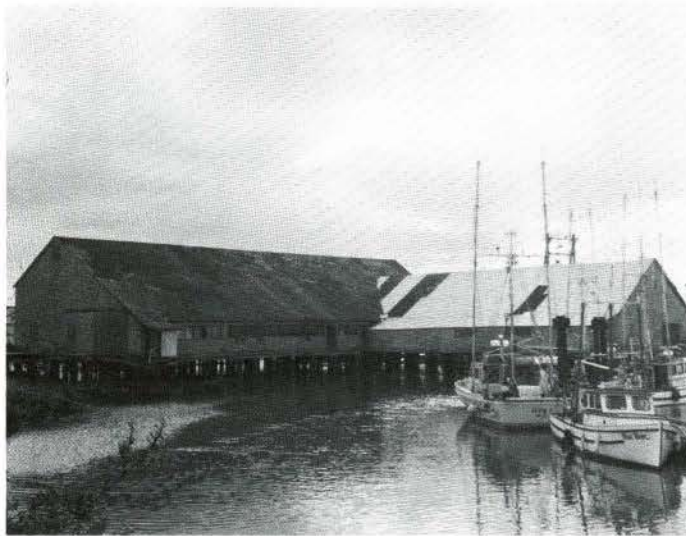
Figure 6. Pacific Coast Cannery as it looked in 1983. The "L" configuration common to pre-1900 canneries is clearly seen in this photo.
