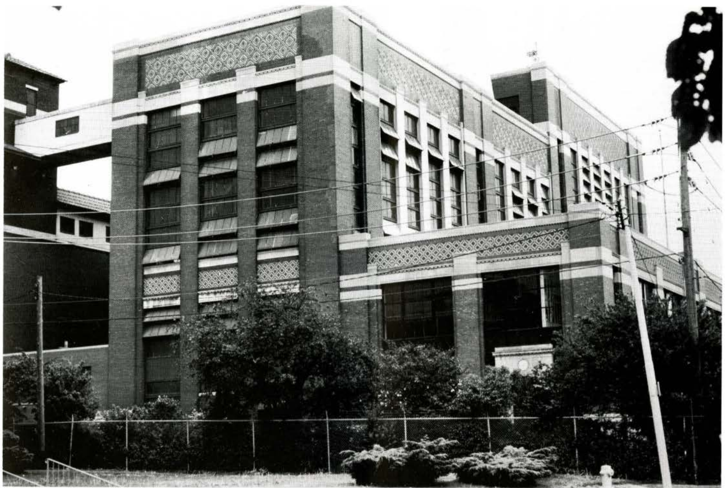
Fig. 9. Details of brickwork, Ford Motor Co. power house (1922-23).
