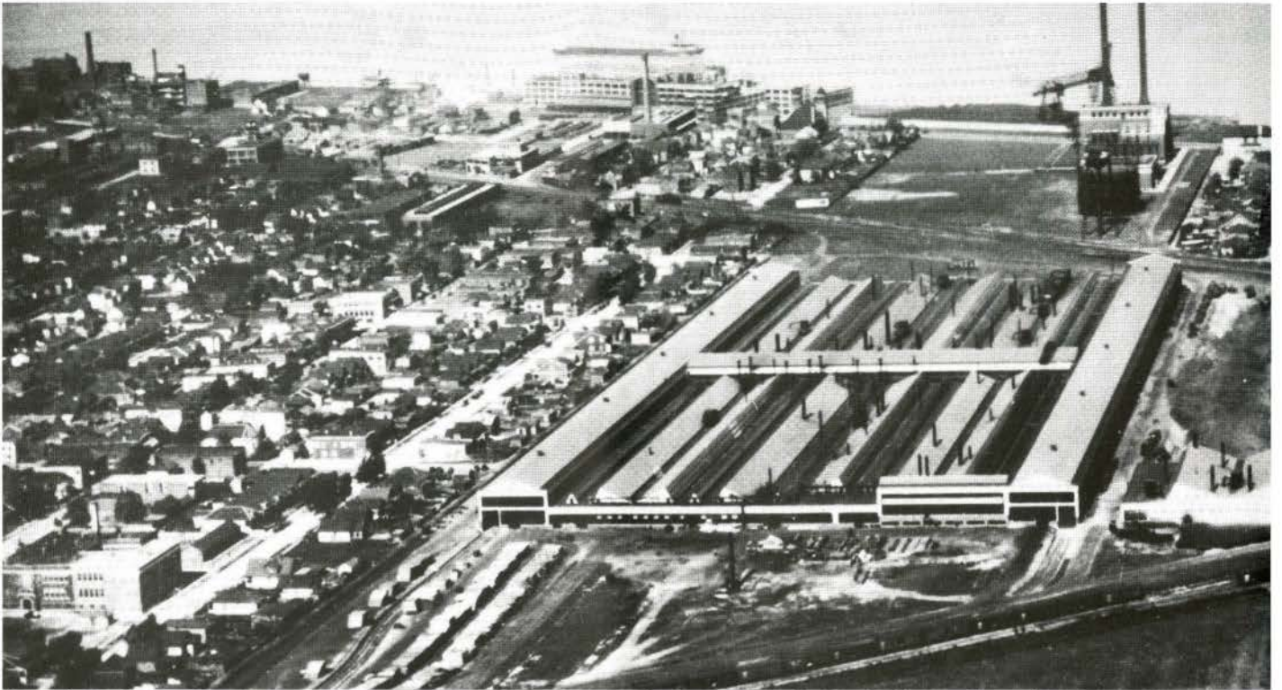
Fig. 8. The Ford Motor Co. factory complex at East Windsor, Ontario, circa 1925. Kahn designed the multi-storey buildings on the riverfront (1910-18) the power house (1922-23) and the engine plant (1923). The latter building, of steel-frame construction, covered a floor space of nearly one million square feet.
