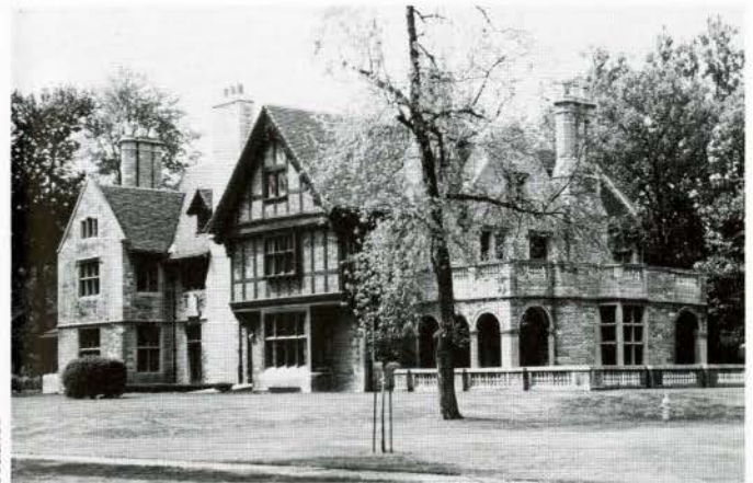
Figure 2. 'Willstead', Walkerville built in limestone, wood and brick filling for E. Chandler Walker in 1905.
