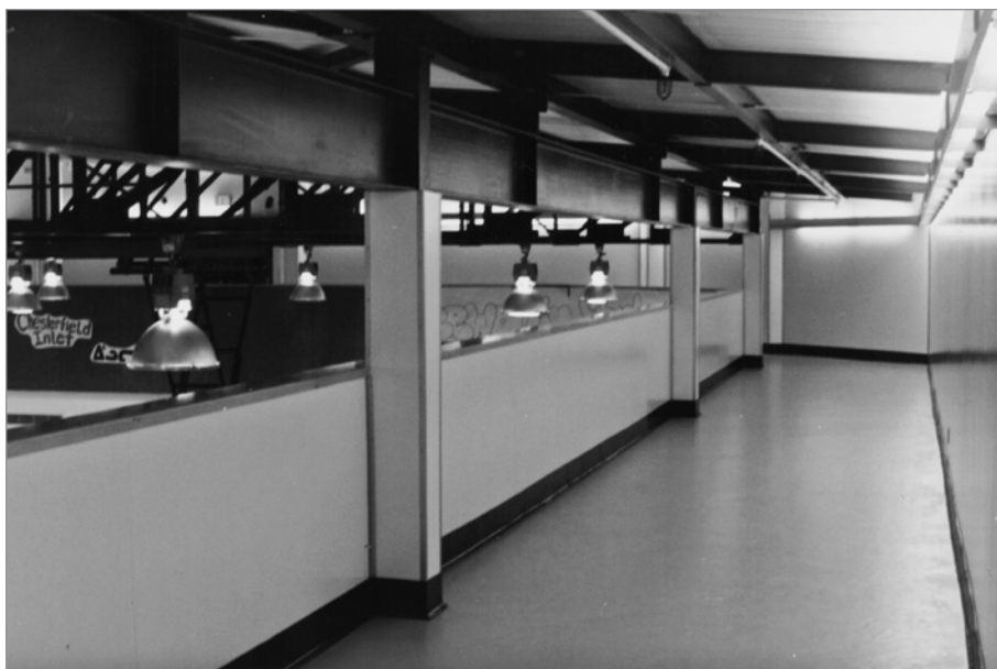
FIG. 19. MAANI ULUJUK, 1982, ELEVATED CORRIDOR AROUND GYMNASIUM. | CLIVE CLARK.
