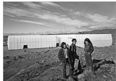
FIG. 10. GORDON ROBERTSON EDUCATION CENTRE, PAPINEAU, GÉRIN-LAJOIE, LEBLANC, EDWARDS, 1971. | REPRODUCED FROM PGL ARCHITECT, ARCHITECTURE DE PGL 1959-1975, MONTRÉAL, 1975 (N.P.).
