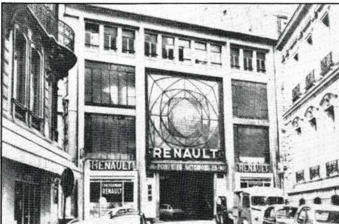
Figure 7. Garage in rue Ponthieu, Auguste Perret, 1905. (Photo: L. Benevolo, History of Modern Architecture (Cambridge, Mass., 1971), p. 325)
