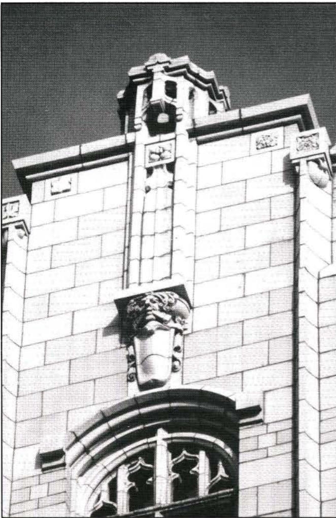
Figure 13. Southeast corner: rooﬂine turret, human head with ribbon, and window tracery, Whalen-Hydro Building, 1987. (Photo: Ray Baker)
