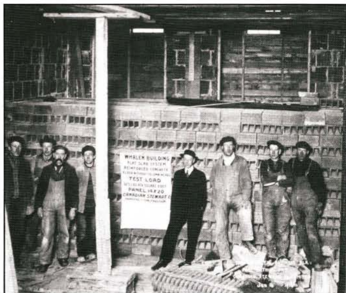
Figure 3. Test load of the reinforced concrete flat slab system at 325 pounds per square foot, 14 January 1914. (Whalen Archives, Norman M. Paterson Library, Lakehead University)
