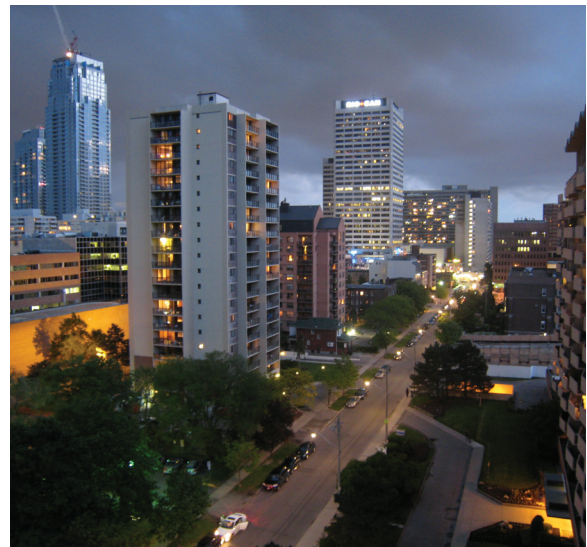
Figure 24. Towers in the park; photograph from Panoramio
