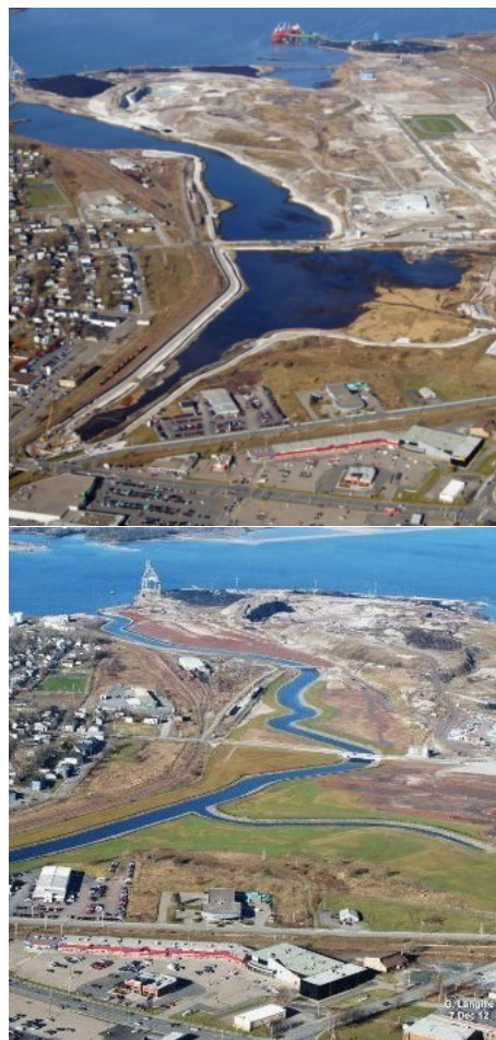
Before and after comparison of the former steel plant site. Top: Sydney tar ponds before remediation; bottom: Sydney tar ponds after remediation; image taken from AECOM Transforms Contaminated Site in Canada into Urban Park .
