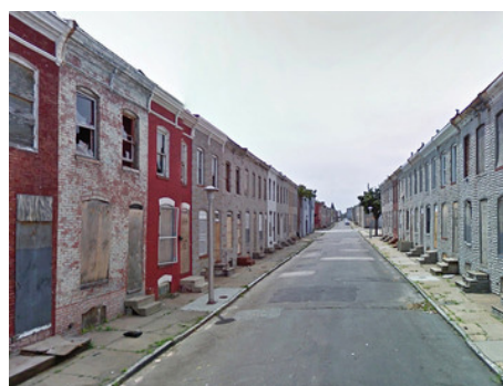
Abandoned rowhouses in Baltimore, Maryland; photograph by Nick Barrickman, from The Deindustrialization of Baltimore .
