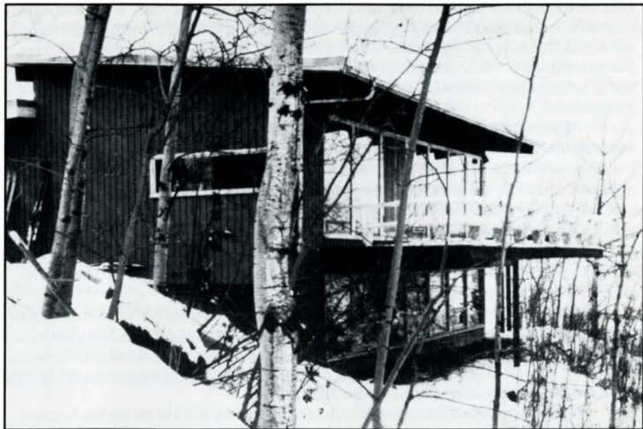
Figure 2 (above). Side view of Wallbridge and Imrie's home and office, Six Acres. The main living areas on the ground floor and the offices and spare bedroom in the basement face the ravine. (Provincial Archives of Alberta)
