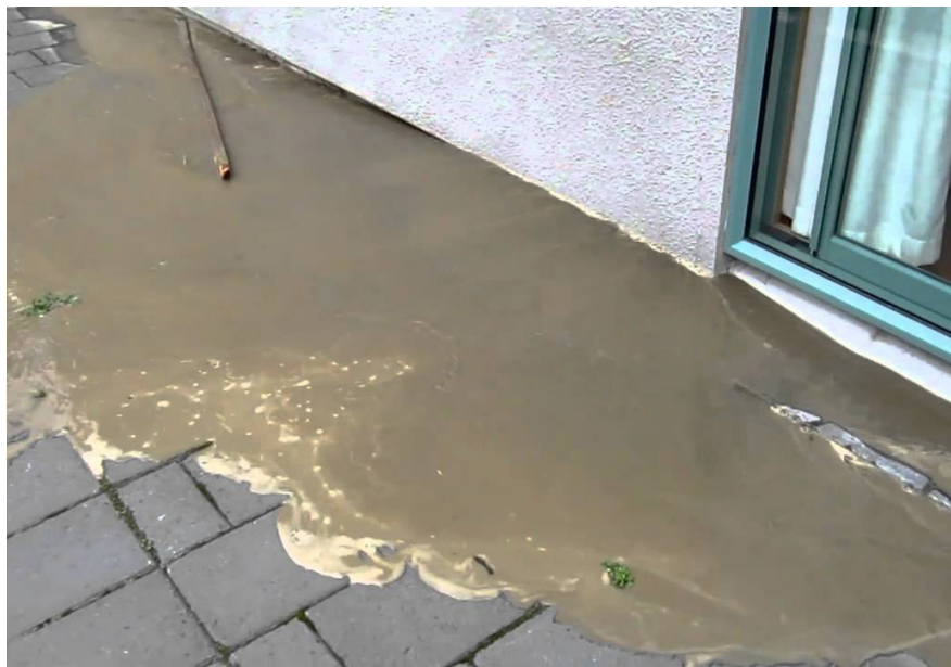
Figure 15. House sinking into the liquefied soil, 2011; from Christchurch City Libraries.
