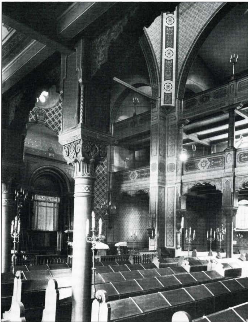
Fig. 2. Interior, Dresden Synagogue, Germany. (Krinsky, Carol Herselle. Synagogues of Europe: Architecture, History, Meaning . Cambridge, Massachusetts: The MIT Press, 1985, p. 279)
