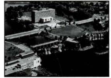
Fig. 41. Aerial view from early 1960s. (City of Ottawa Archives, CA-2478)
