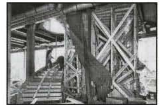
Fig. 35. Construction of the main stairwell, ca. 1957-1958. (City of Ottawa Archives, CA-15206)
