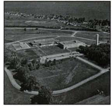
Fig. 39. Northern Electric Research and Development Laboratories, Ottawa, Ontario; constructed, 1960-1963; Bland/LeMoyné/Edwards and Charles Elliott Trudeau, architects. ( Journal of the Royal Architectural Institute of Canada 40, 3 [March 1963], 46)
