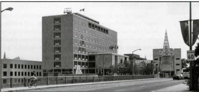
Fig. 4. View of the former Ottawa City Hall from the northeast side, across Sussex Drive. (A. Waldron, HSB, 2001)
