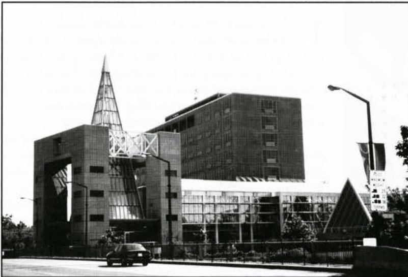
Fig. 3. View of the Bytown Pavilion and original slab block from the northwest, across Sussex Drive. (A. Waldron, HSB, 2001)
