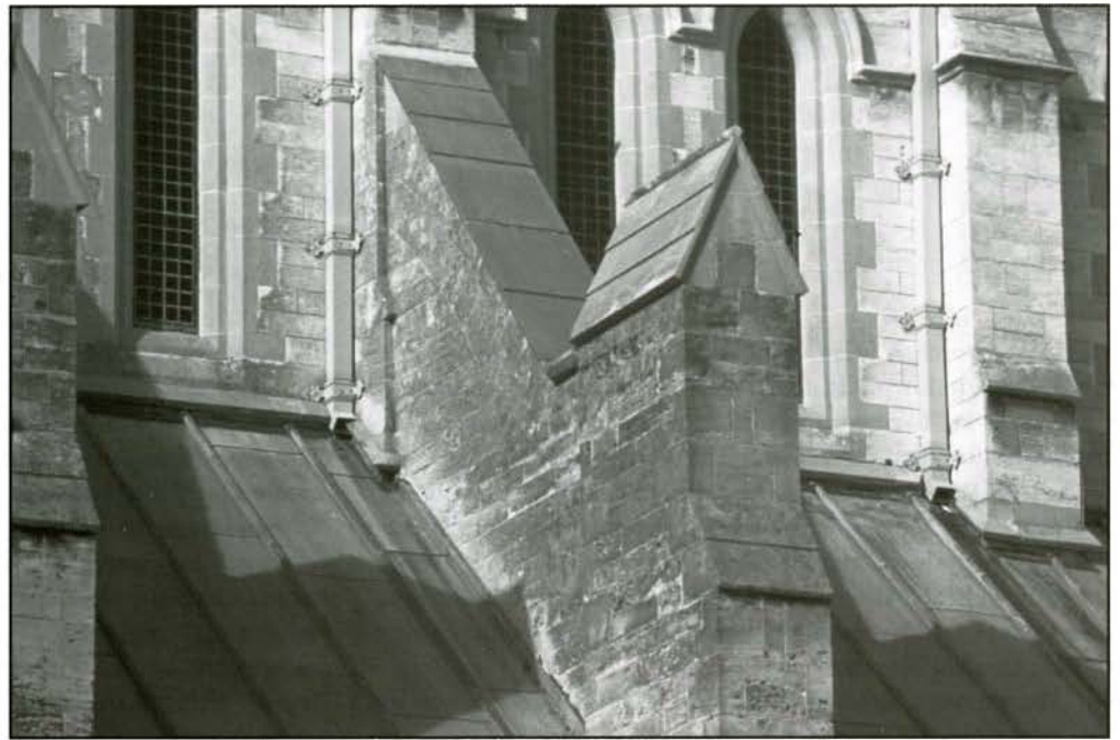
Fig. 11. Trinity Church, Bermuda. Reinforcements above the aisle. (Photo: Barry Magrill)
