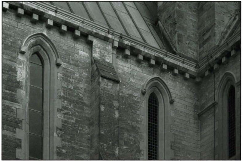
Fig. 9 Trinity Church, Bermuda. North transept showing carved and uncarved window labels. (Photo: Barry Magrill)
