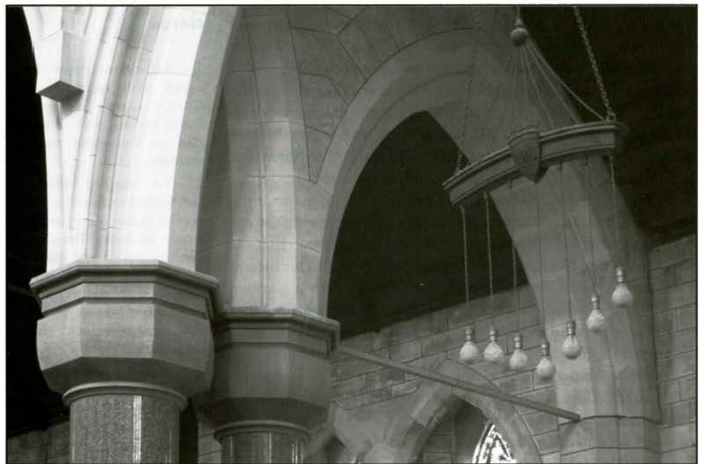
Fig. 12. Trinity Church, Bermuda. Main arcade, twinned columns with transverse arch and arch segment in the aisle. (Photo: Barry Magrill)
