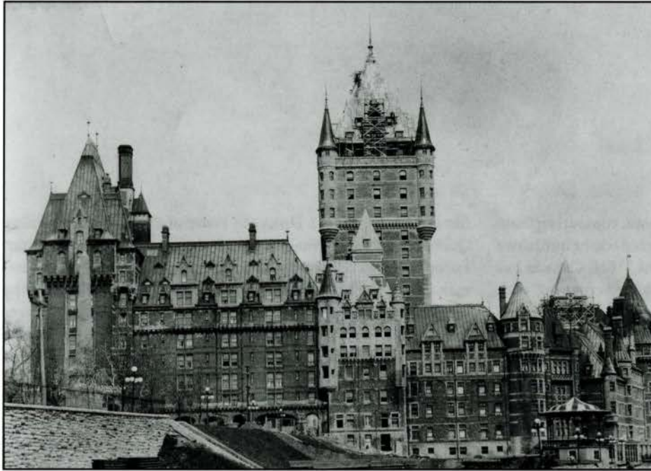
Fig. 16. «Dufferin Terrace and the Chateau Frontenac, new tower under construction, Québec City.» Edward and W.S. Maxwell, architects 1920-1924. (Notman Photographic Archives, McCord Museum of Canadian History, MP-0000.2078.4)
