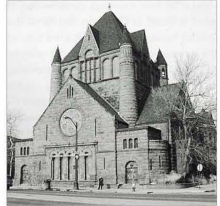
FIG. 12. FIRST PRESBYTERIAN CHURCH, DETROIT, MICHIGAN, 1889-91, GEORGE D. MASON (ARCHITECT) – EXTERIOR. | CANDACE IRON
