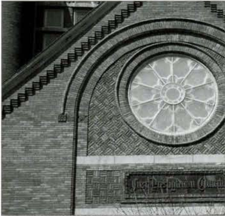
FIG. 4. FIRST PRESBYTERIAN CHURCH, CHATHAM – EXTERIOR DETAIL. | MALCOLM THURLBY
