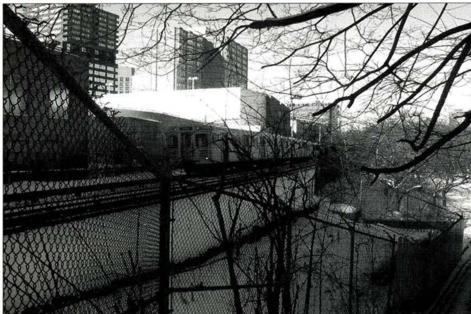
FIG. 21. VIEW OF THE STUDIO BUILDING FROM SEVERN STREET. | ANDREW WALDRON, PARKS CANADA, 2004
