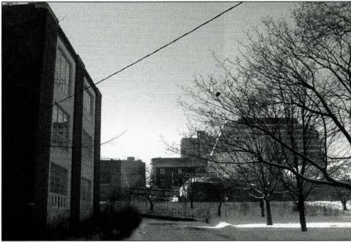
FIG. 21. VIEW OF THE STUDIO BUILDING FROM SEVERN STREET. | ANDREW WALDRON, PARKS CANADA, 2004
