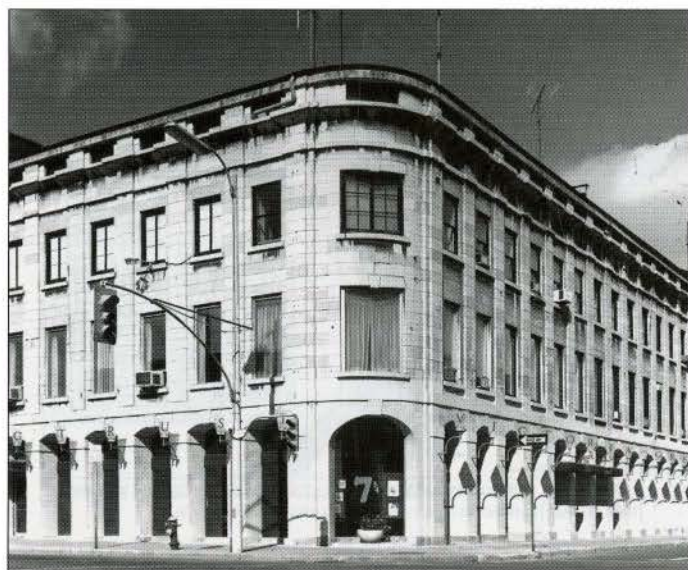
FIG. 10. WILSON'S BUILDINGS (NOW BANK OF NOVA SCOTIA), KINGSTON, BY GEORGE BROWNE, 1841-1842. | JOHN BREBNER
