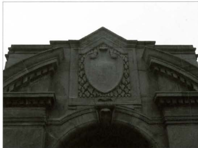
FIG. 10. DETAIL OF THE ORNAMENTAL STONework AT THE TUNNEL PORTAL PEDIMENT. | STEVEN MANNELL
