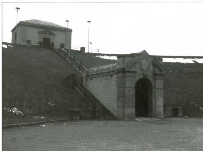
FIG. 9. VIEW OF THE VALVE HOUSE (UPPER LEVEL) AND TUNNEL PORTAL (LOWER LEVEL) AT THE CROOK OF THE RESERVOIR. | STEVEN MANNELL
