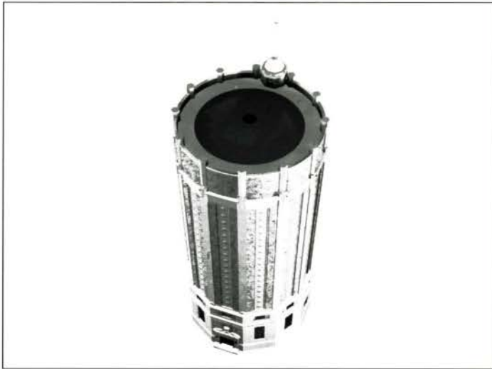
FIG. 1. THE TOWER OF PURE WATER: DIGITAL RECONSTRUCTION OF THE UNBUILT DISTRICT NO. 3 OVERHEAD TANK, VIEWED FROM ABOVE SHOWING THE FRONT FAÇADE OF THE TANK FACING THE PLAYING FIELDS ON TOP OF THE ST. CLAIR RESERVOIR. THE DOORWAY WITH BROKEN PEDIMENT AND MONUMENTAL URN IS AT THE BASE; THE ROOFTOP CUPOLA ACCOMMODATES THE ROOF ACCESS LADDER. | RENDERING AND DIGITAL MODEL: BENJAMIN CHECKWITCH, STEVEN MANNELL, WILLIAM RAWLINGS
