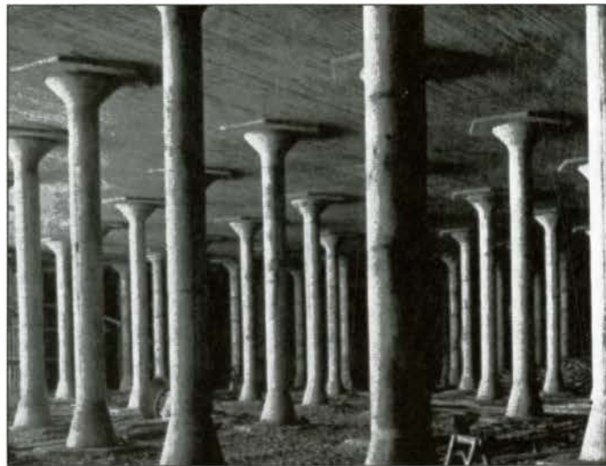
FIG. 8. VIEW OF INTERIOR OF RESERVOIR UNDER CONSTRUCTION, SHOWING HEXAGONAL COLUMN GRID. | PHOTO: ARTHUR GOSS, CITY OF TORONTO ARCHIVES, RGB, SERIES 65, ITEM 81
